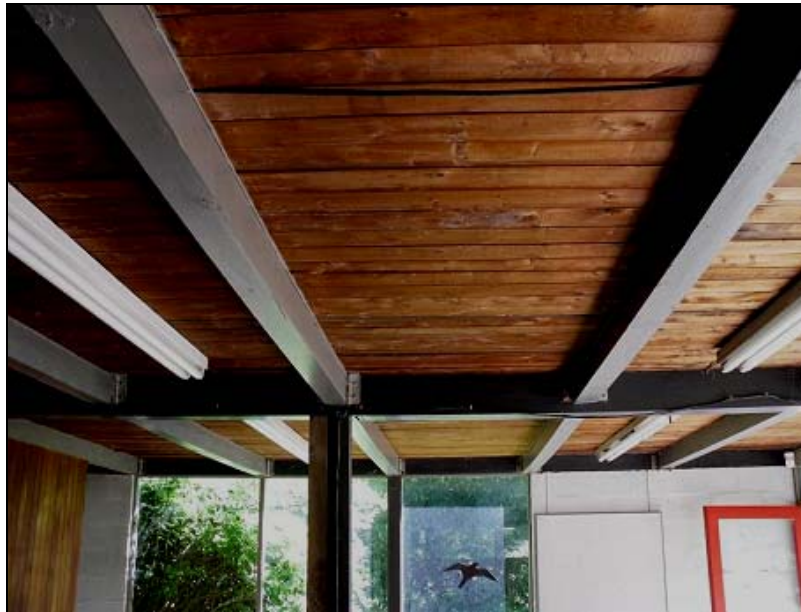
5.5.4 , Interior Looking East, Ceiling Frame & Deck, June 2010.
