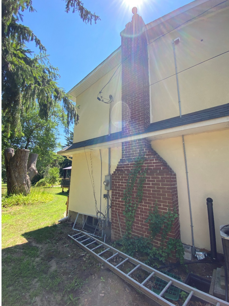
Figure 6 The north façade of 2230 Mississauga Road. (Photo from client.)
