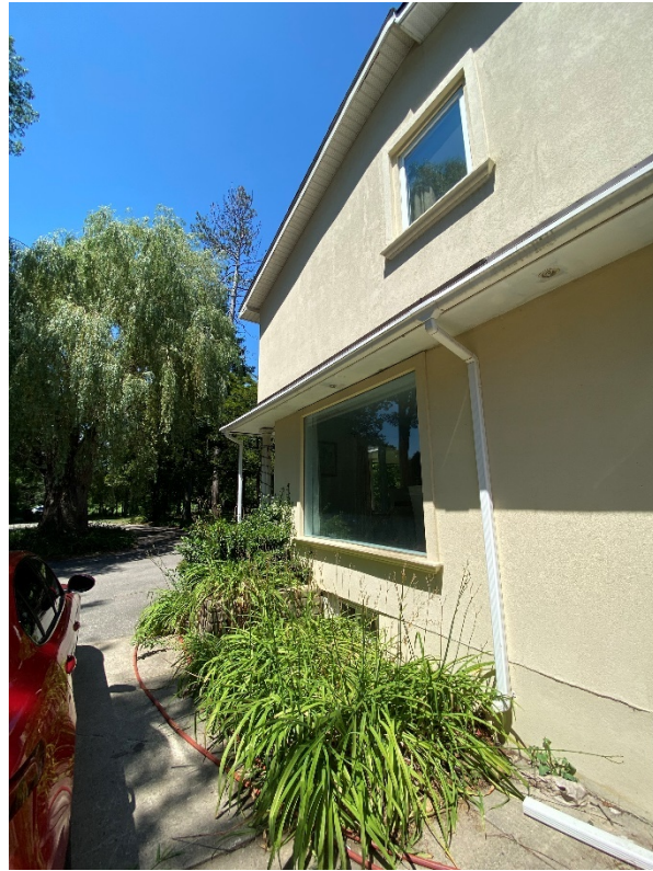
Figure 4 The south façade of 2230 Mississauga Road, Mississauga. (Photo from client.)
