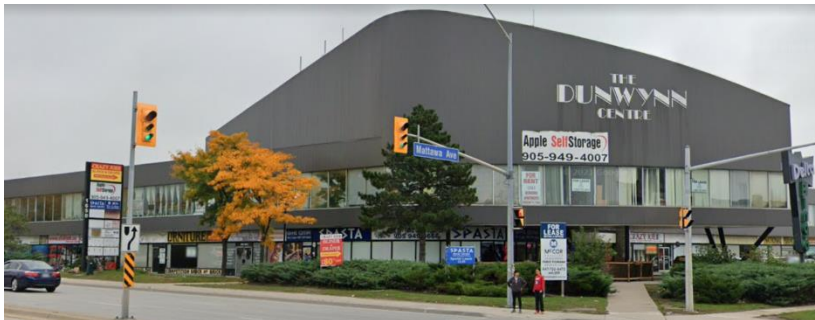
Existing Conditions – facing southeast on Dundas Street East
