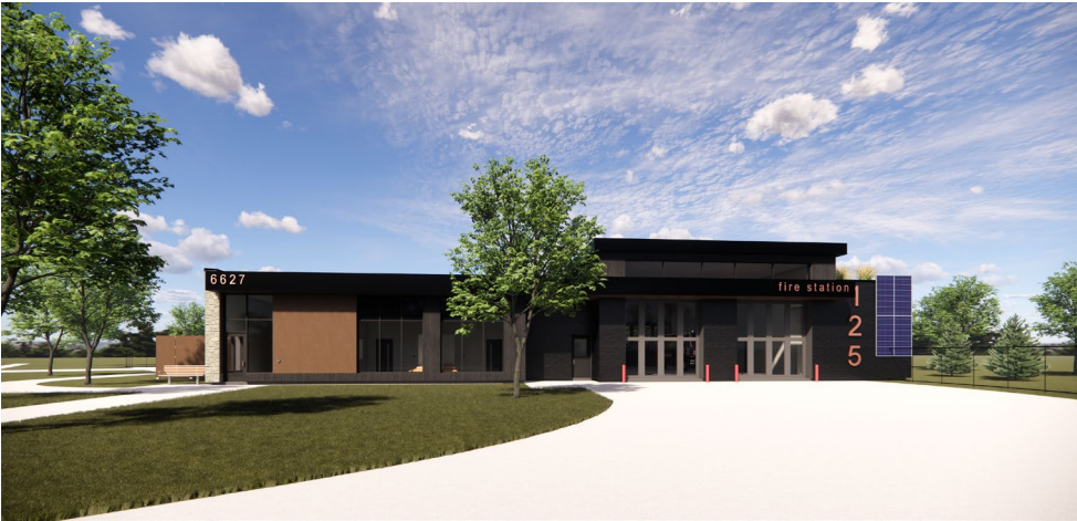
Fire Station 125 (City's First Net Zero Building)
