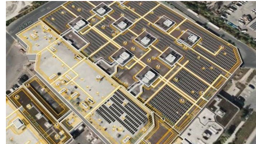
Solar Panels to be Installed on 975 Central Parkway Transit Facility
