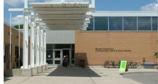
South Common Community Centre and Library
