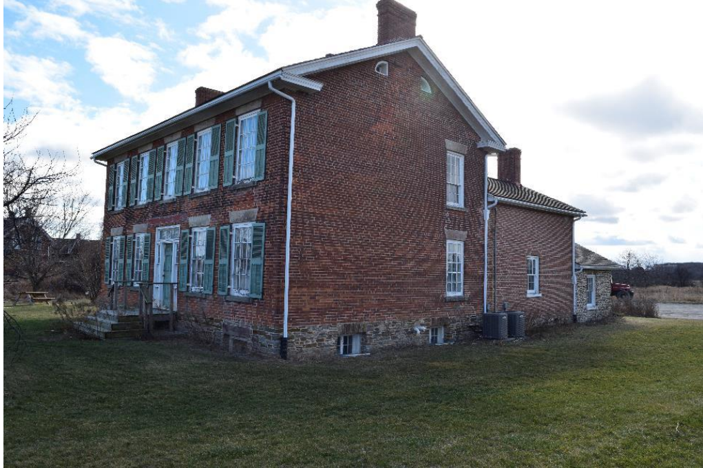
Image 17: Northwest exposure of Gardner-Dunton House.
