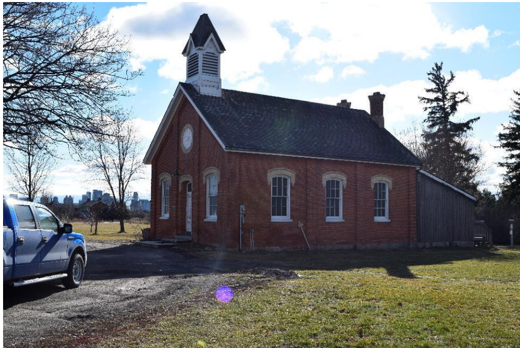
Image 1: Northwest exposure of Britannia School House.
