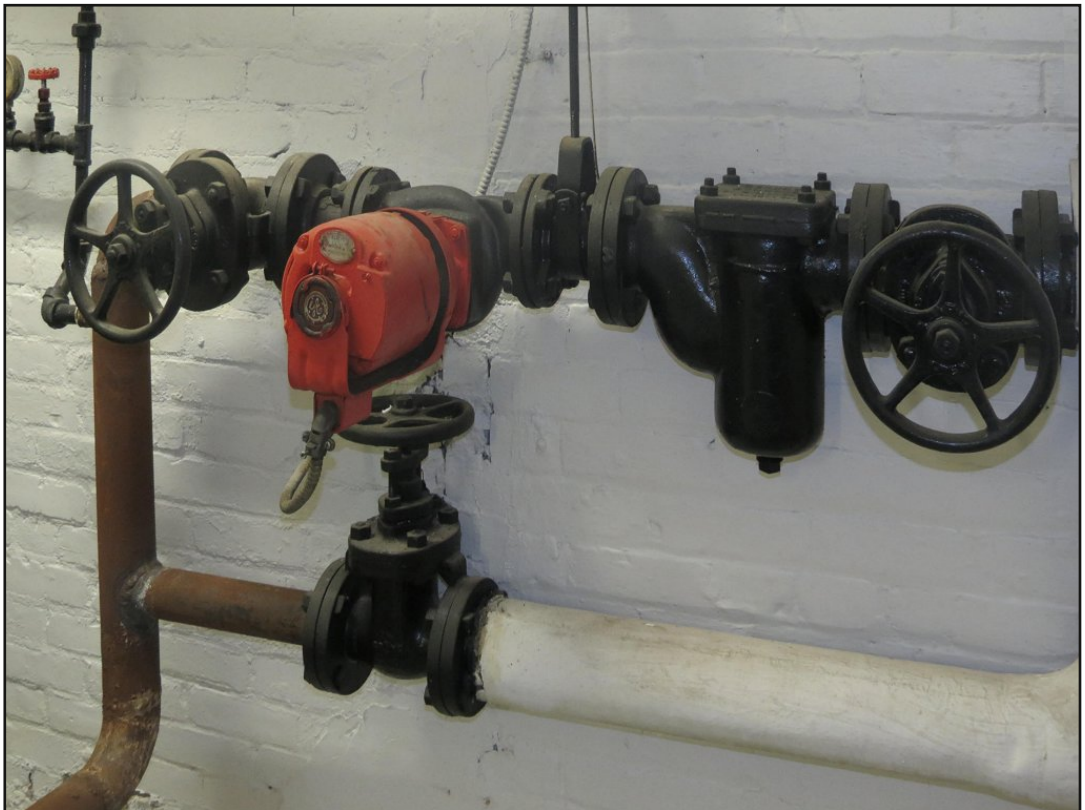
2.3.2z: modern and 1923 water control valves
