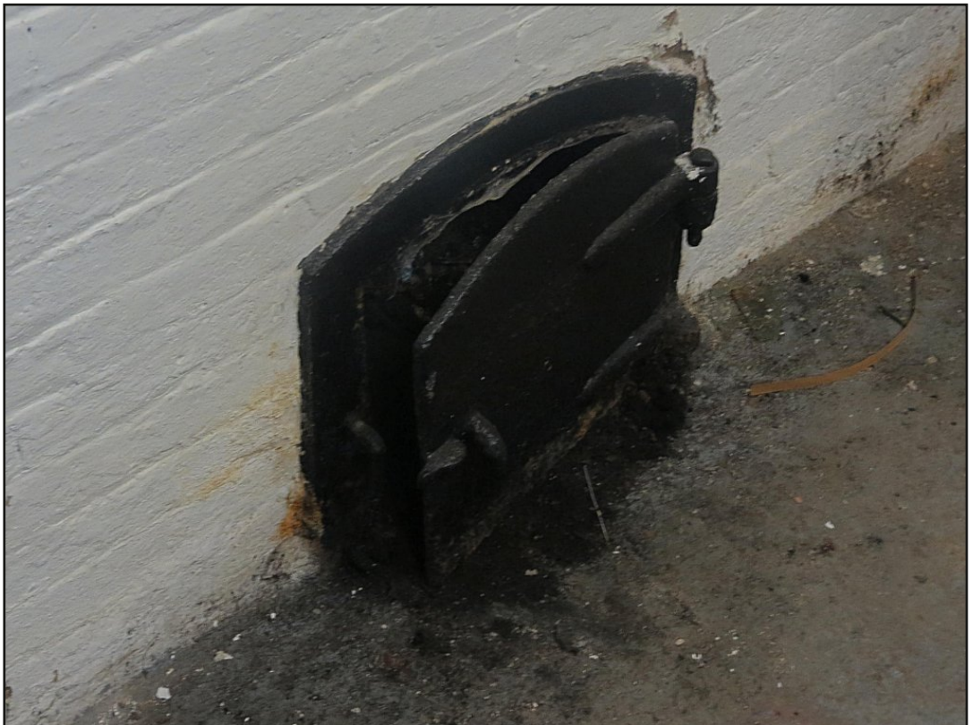
2.3.2x: coal chute outlet
