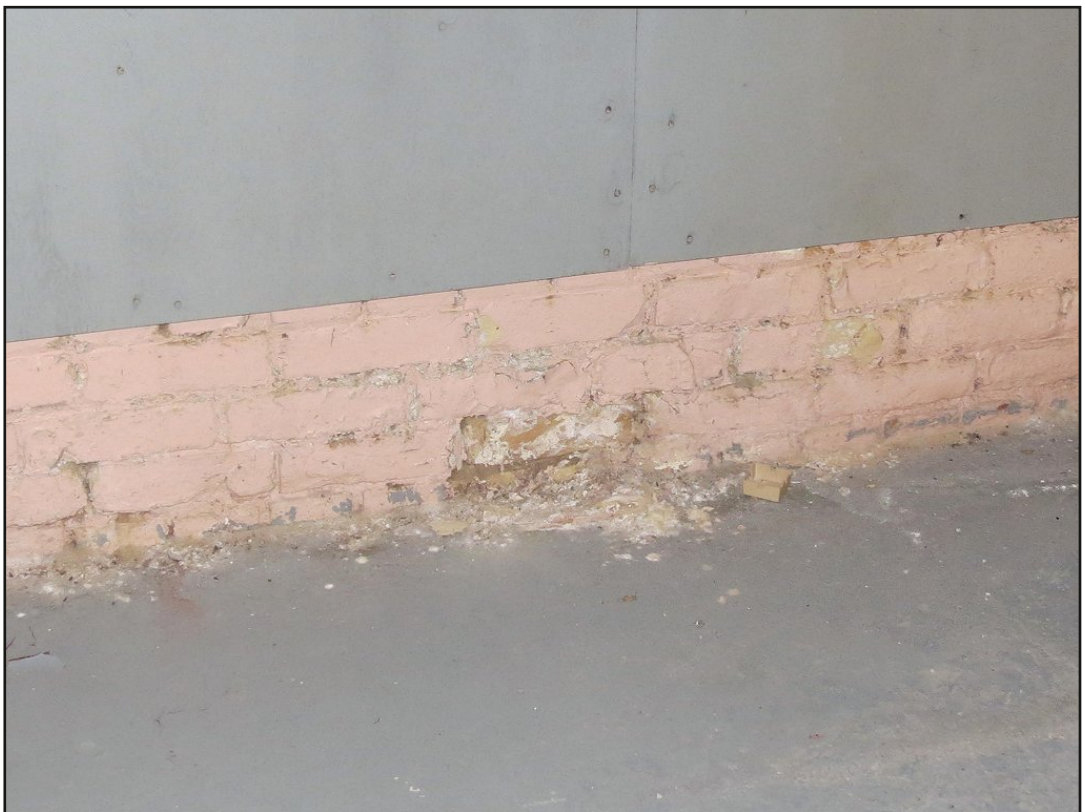
2.3.2l: deteriorating bricks, basement
