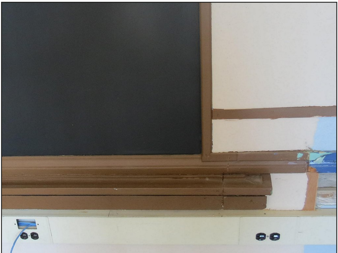
2.3.2h: evidence of the lengthened chalkboard, and outlets for computers
