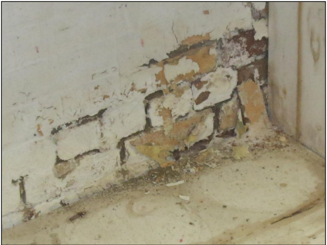
2.3.2k: deteriorating bricks, basement
