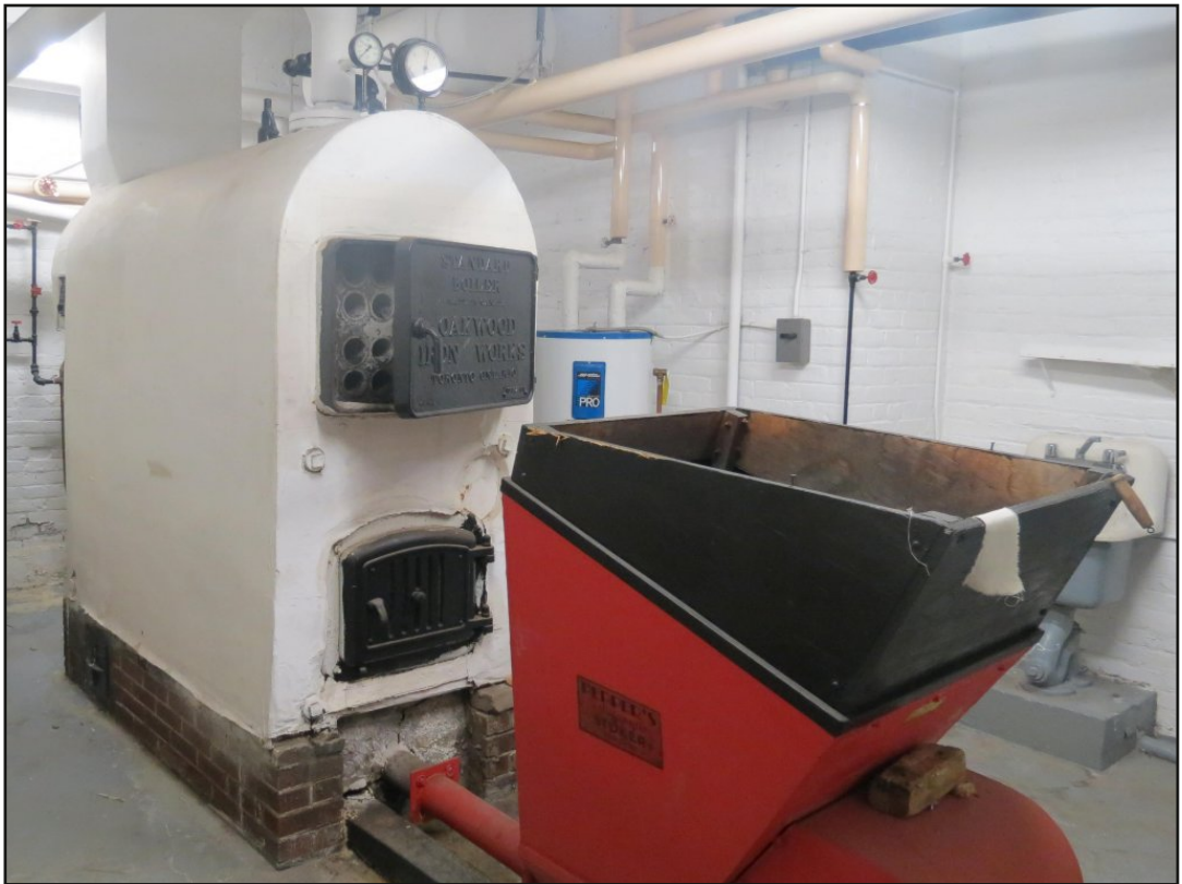
2.3.2s: boiler and coal scuttle
