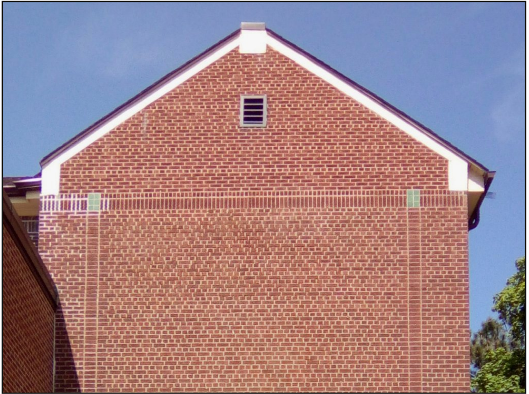
2.3.1h: variations in brick bonds, west elevation of 1923 section
