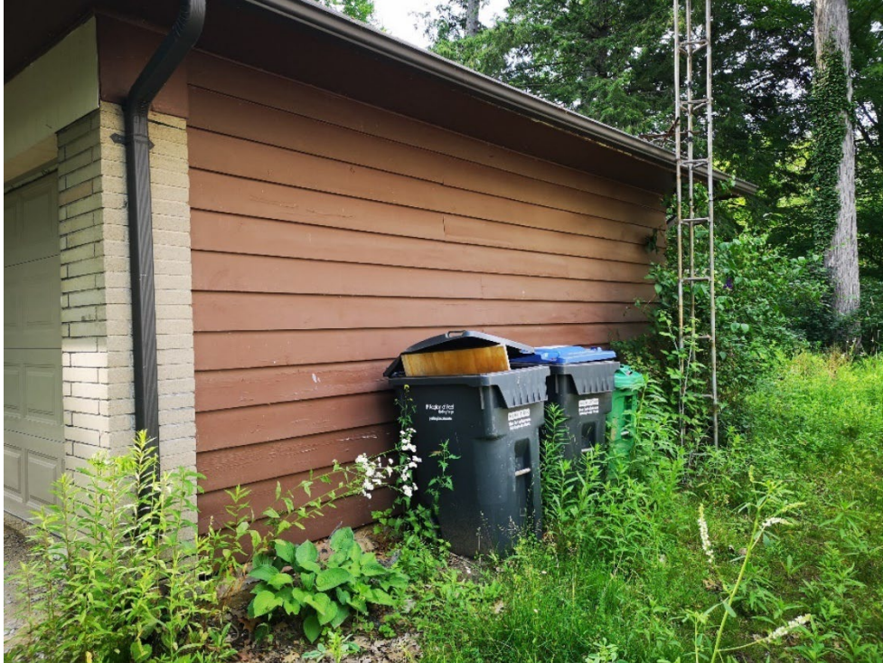
SOUTH ELEVATION. NOTE WOOD SIDING
