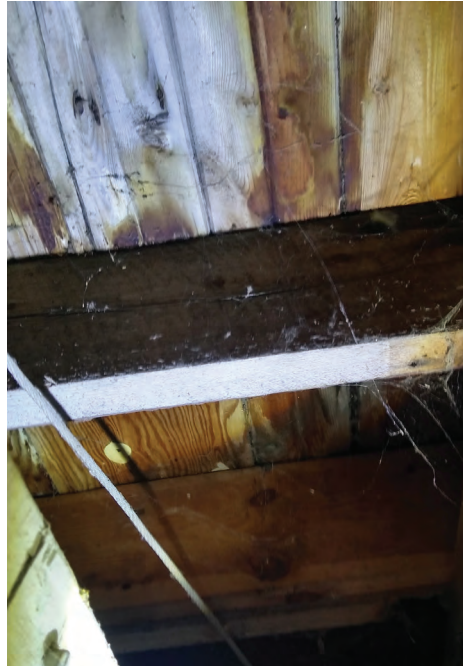
Signs of water damage of the attic floor. Source: ATA Architects Inc. (2023)
