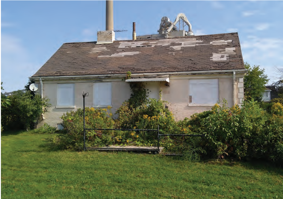
Photo of the front of the house. Asphalt shingle gable roof and brick walls. The structure is on and a half storeys in height with a basement. The entrance is slightly off centre. Source: ATA Architects Inc. (2023)
