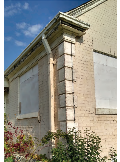
Details are made from wood including a decorative bed molding and frieze board and faux quoining at the corners. Source: ATA Architects Inc. (2023)
