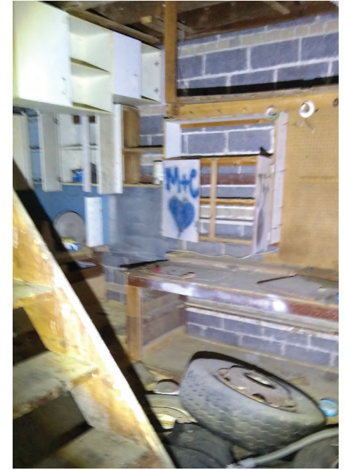
Interior face of walls appear to be block unit masonry. Source: ATA Architects Inc. (2023)
