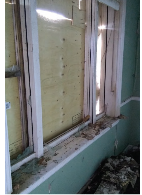
Windows have been smashed through out the building. None appear to remain intact. Source: ATA Architects Inc. (2023)
