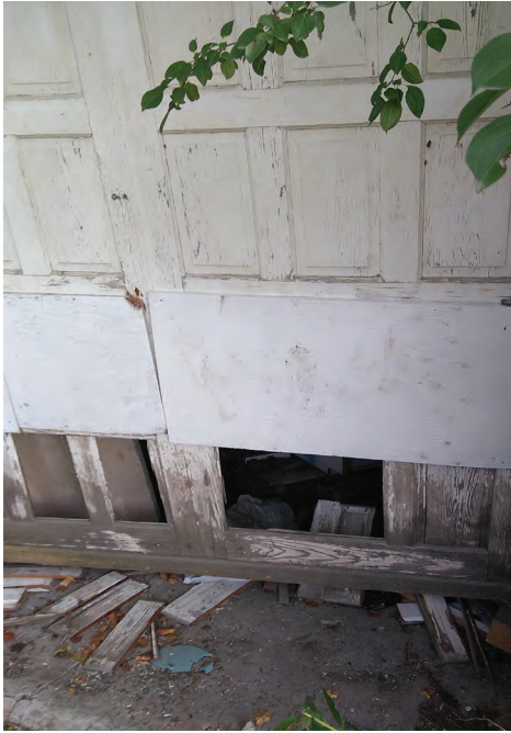
Garage door was broken and inoperable Source: ATA Architects Inc. (2023)
