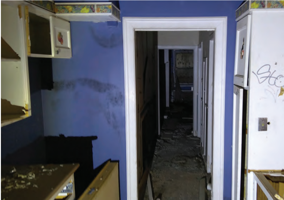
Interior, kitchen looking down the hall to the front room of the house. Signs of extensive damage and vandalism continue through this space along with signs of mold. Source: ATA Architects Inc. (2023)
