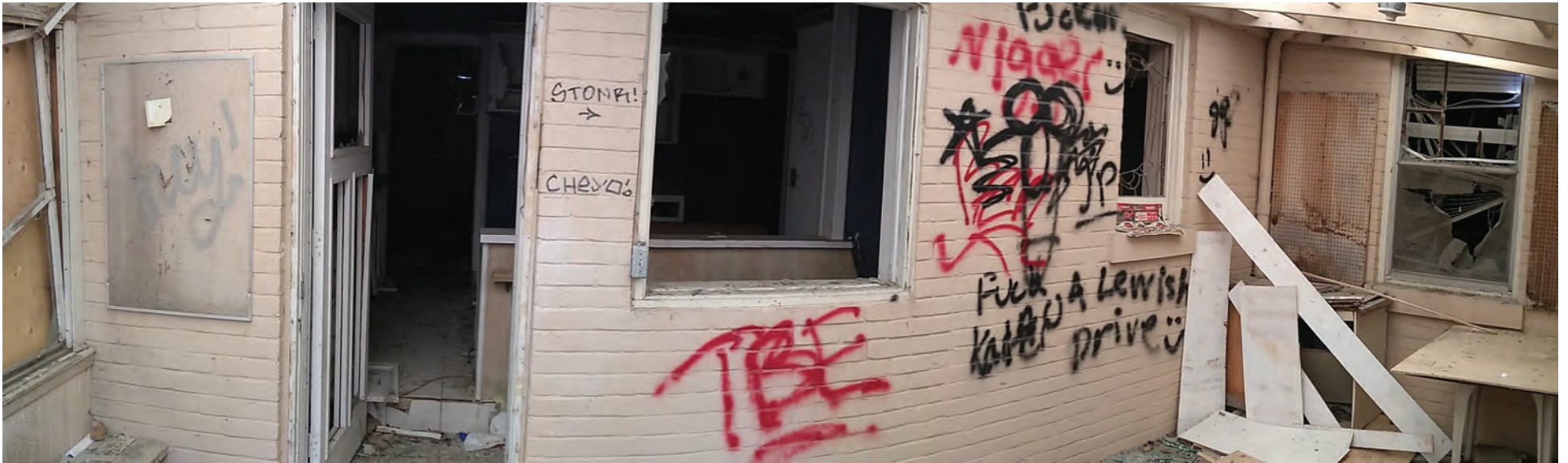
Interior of the enclosed porch. All of the windows have been smashed, extensive graffiti on the walls and other vandalism. Source: ATA Architects Inc. (2023)
