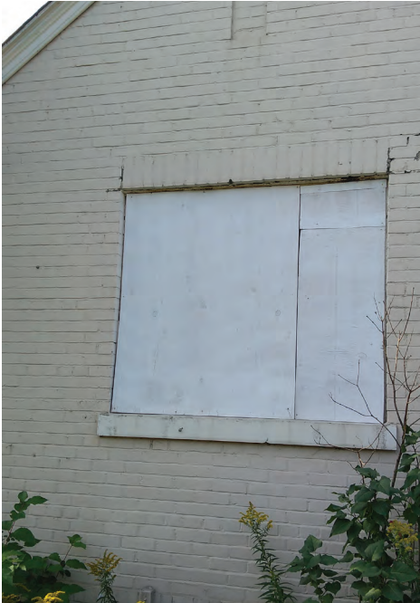
Brick soldier courses are located above some of the windows. Sills have been clad in aluminum. Source: ATA Architects Inc. (2023)
