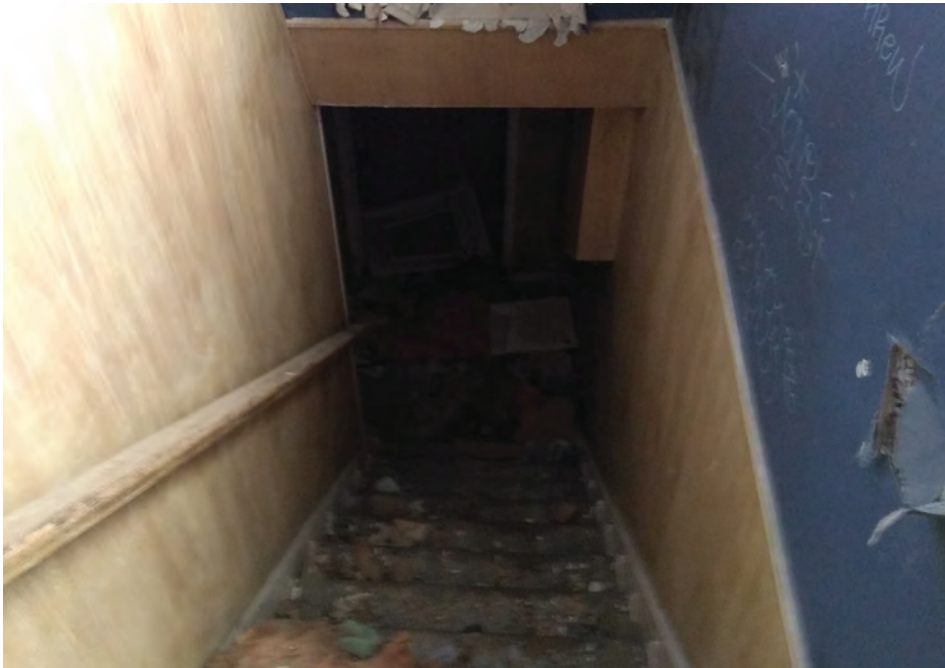
Stairs leading from the kitchen to the basement. Stairs are in a fragile condition, one broke under the weight of the reviewer during the site visit. Source: ATA Architects Inc. (2023)
