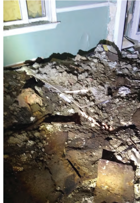
Debris from collapsed ceiling, significant mold growth present. Source: ATA Architects Inc. (2023)
