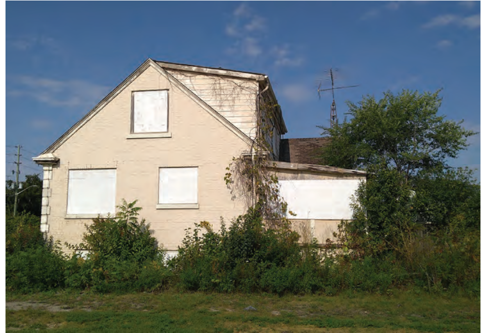
View of the southwest elevation. An enclosed porch addition on the ground floor can be seen. Also a shed dormer can be seen above. Window openings vary in size through the building. Brick soldier courses are visible above some windows. Source: ATA Architects Inc. (2023)
