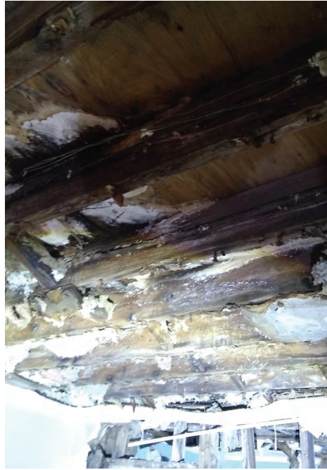
Ceiling had completely collapsed in the front room. Structure and floor boards of the floor above were visible. Clear signs of significant water damage and rot was visible. Reviewer did not proceed to second floor due to safety concerns related to the structural integrity of the floor. Source: ATA Architects Inc. (2023)
