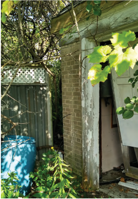
Garage appears to be brick face with a concrete block structure. Garage door was broken and inoperable. Source: ATA Architects Inc. (2023)
