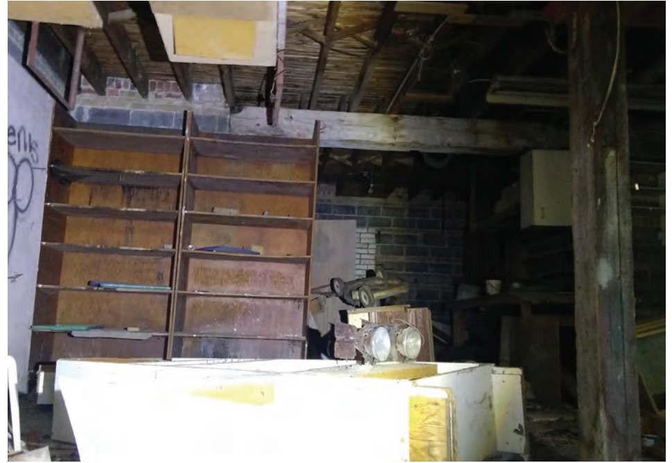
Interior of garage also appears to have been vandalized. Wood post and beam structural supports are visible. Source: ATA Architects Inc. (2023)
