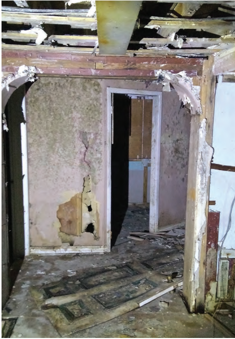
Basement condition similar to the first floor. Advanced state of decay and damage. Ceilings have been removed. Extensive water damage and mold growth. Source: ATA Architects Inc. (2023)
