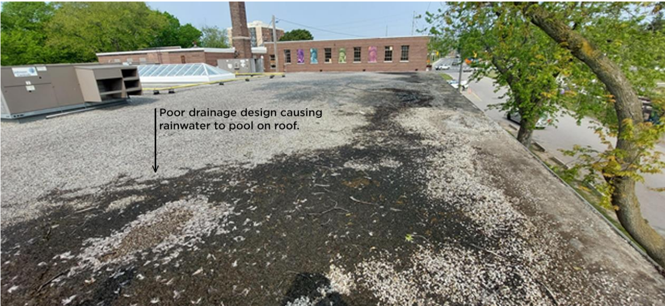
Figure 1. Existing roof condition. Dark areas indicate rainwater pooling as a result of inadequate drainage design.
