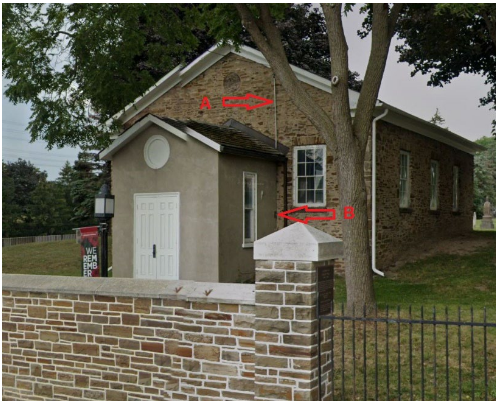
Existing service: A – service stack, B – meter
