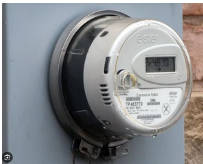
Typical new (exterior mounted) Alectra meter
