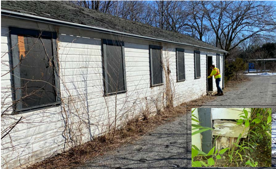
HEADER HOUSE FOUNDATION - the frame building sits directly on a concrete pad foundation - there is significant deterioration around the base of the building because it sits directly on grade and is sited at the base of a slope
