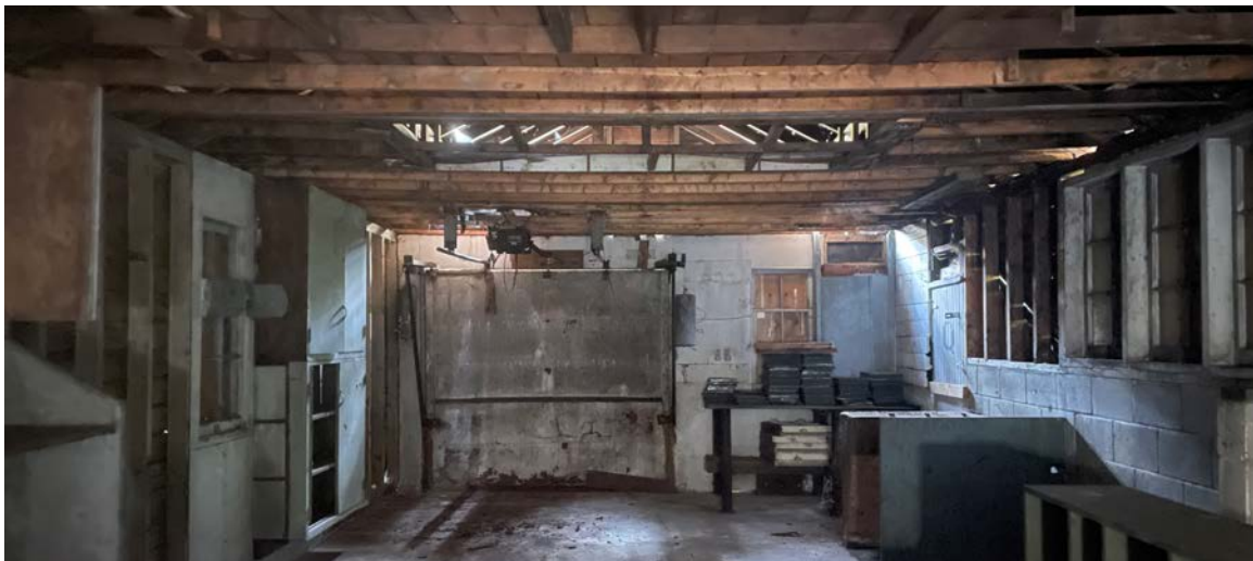
HEADER HOUSE INTERIOR - daylight shining through holes where the roof has collapsed. The roof rafters are rotted and saturated.
