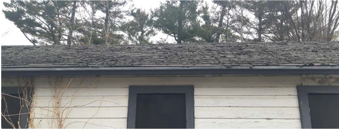
HEADER HOUSE ROOF - deteriorated roof shingles
