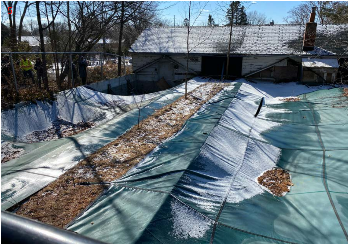
COLD FRAME FOUNDATIONS – temporary tarping installed to prevent water pooling in the exposed foundations
