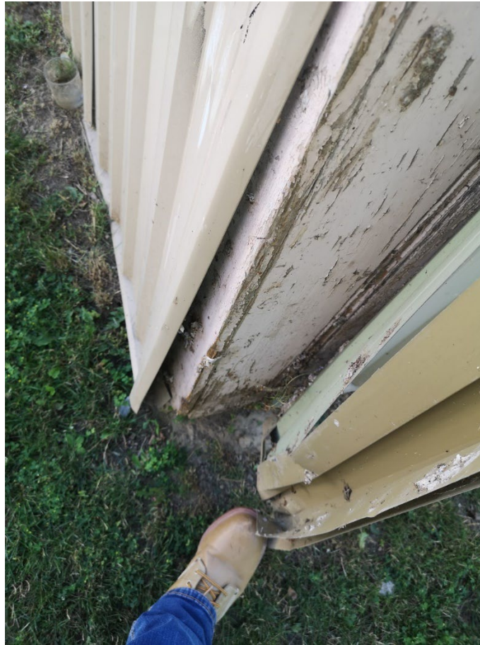
STORAGE BUILDING ORIGINAL WOOD SIDING VISIBLE BENEATH METAL CLADDING
