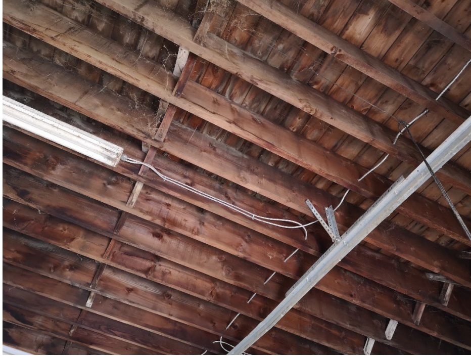
STORAGE BUILDING ROOF STRUCTURE SHOWING ORIGINAL JOISTS AND SHEATHING, NEWER LIGHT FIXTURES, ELECTRIC WIRING AND OVERHEAD DOOR TRACK
