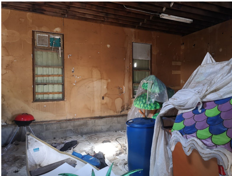
STORAGE BUILDING INTERIOR FACING WEST. NOTE ORIGINAL WINDOW OPENINGS EXTANT WITH REMNANT OF DOUBLE HUNG SASH VISIBLE. BACK OF METAL SIDING PANELS ARE VISIBLE THROUGH THE WINDOWS
