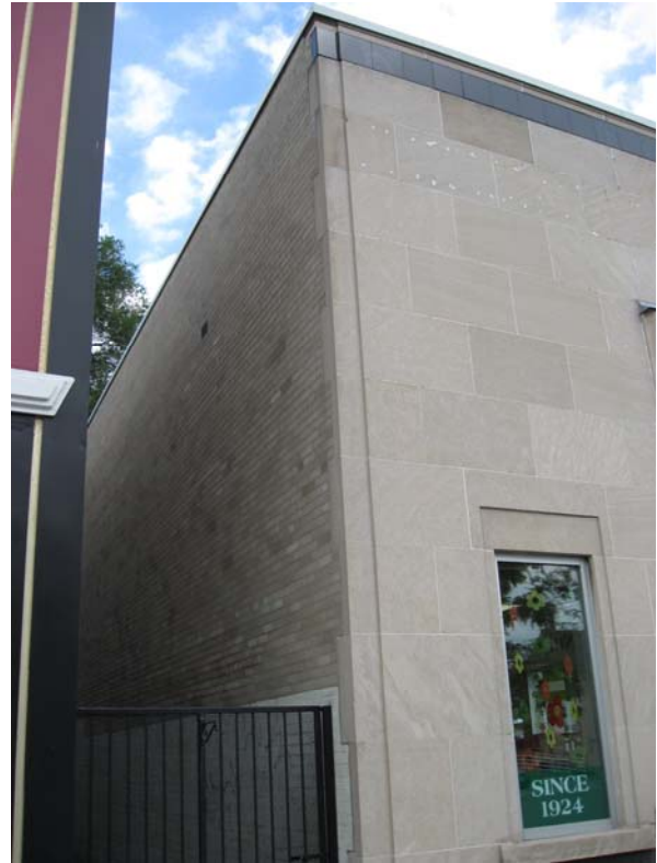
Figure 11: Southwest face, August 2009.
