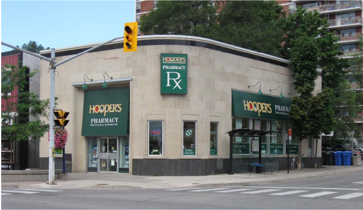
Figure 7: Southeast façade, August 2009.
