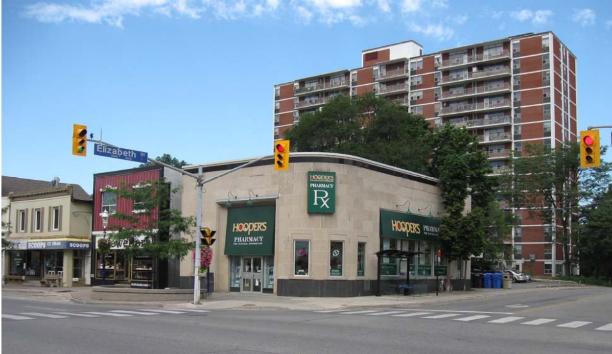
Figure 6: Long shot of southeast façade, August 2009.
