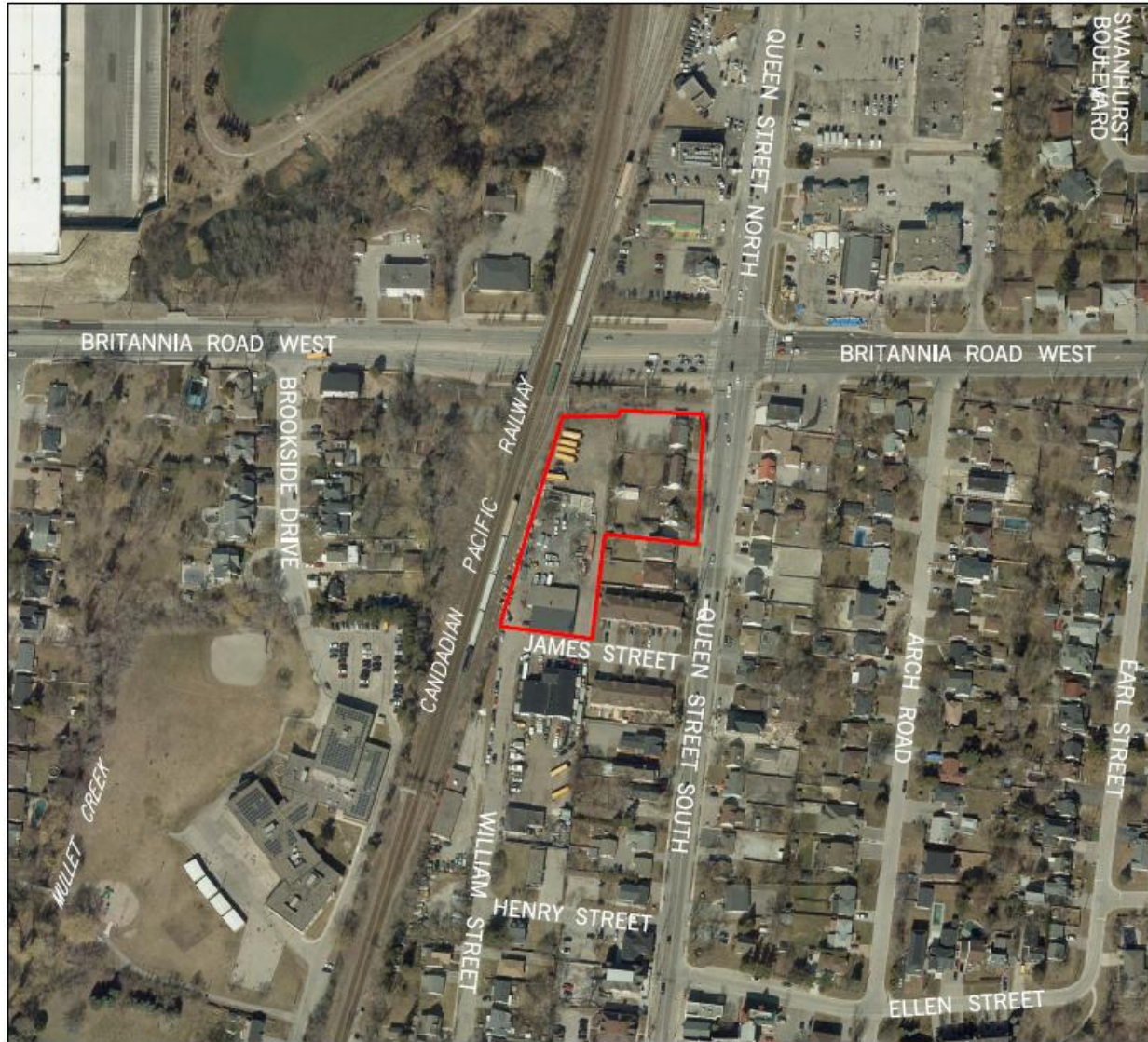
Aerial Photo of 6, 10 and 12 Queen Street South, 16 James Street, and 2 William Street
