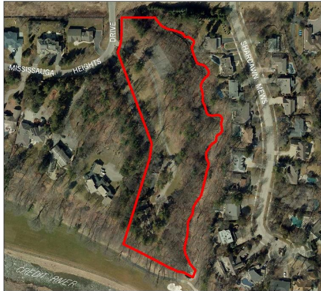
Aerial Image of 900 Mississauga Heights Drive
