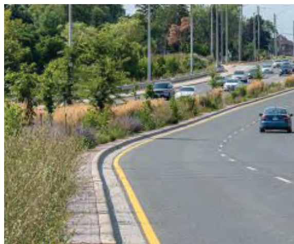
Figure 4.13. The bioswales along Mississauga Road represent the on-going green infrastructure initiatives within the City.
