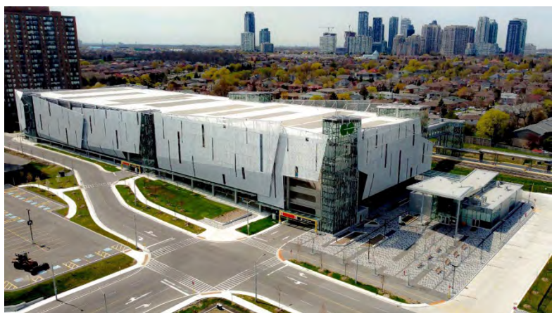
Figure 7.7. Cooksville GO Station's newly constructed package garage supports TDM initiatives by facilitating multi-modal transportation.
