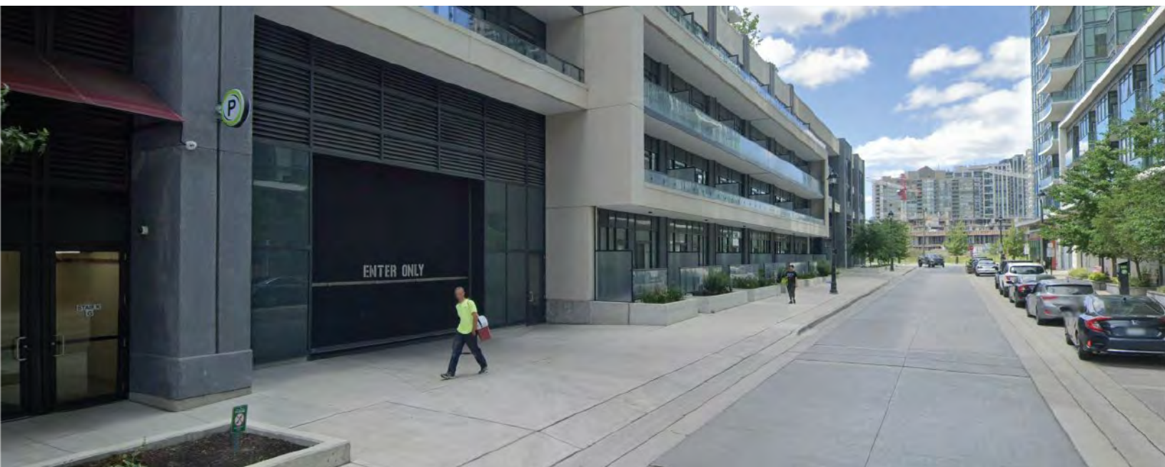
Figure 8.9. Locate high-rise parking entrances at rear of buildings, away from the main street.
