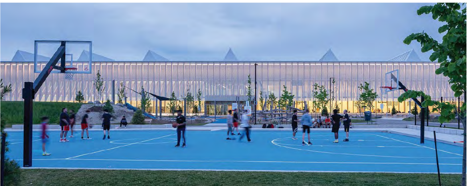
Figure 17.4. Churchill Meadows Community Centre and Mattamy Sports Park is a recreational facility equipped with a variety of amenities and programs.
