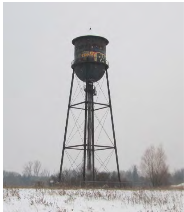
Figure 4. The Water Tower on the Canadian Arsenal Lands is one of the last remaining elements on these lands, dating back to 1910 (c. Hiking the GTA ).
