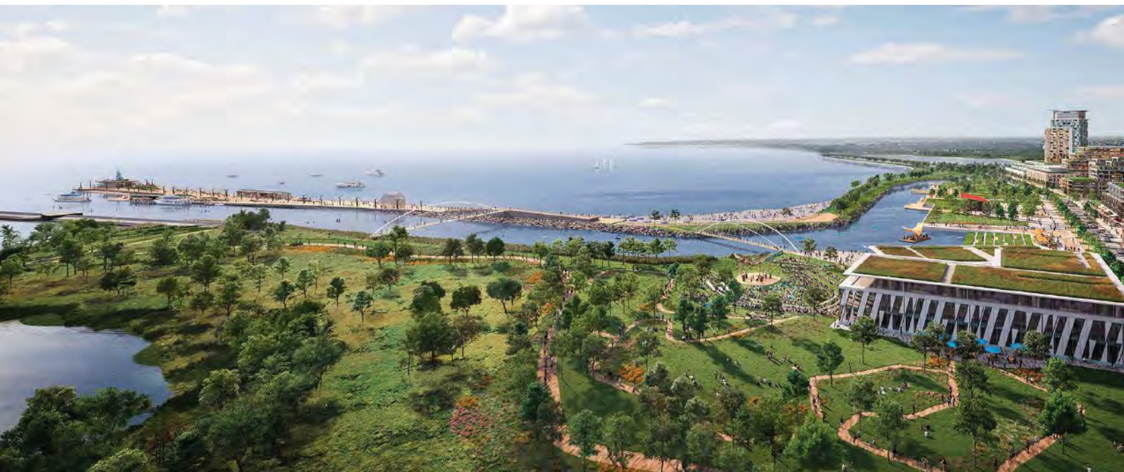
Figure 13.1. A western view of Lakeview Village, overlooking the Jim Tovey Lakeview Conservation Area.
