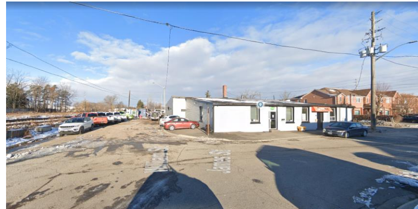
Image of existing conditions fronting James Street
