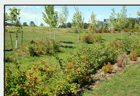
Example of enhanced dry grass swale
