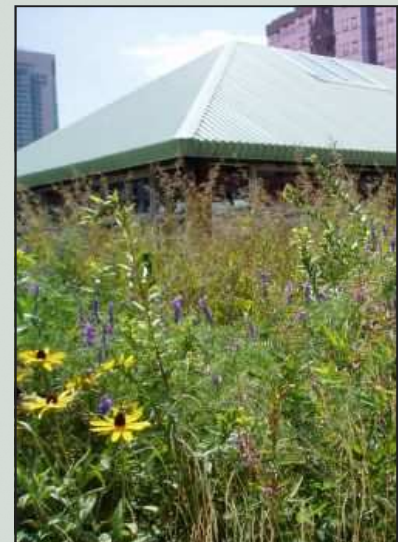
'Intensive' Green Roof sits on parking structure at Mississauga Civic Centre
