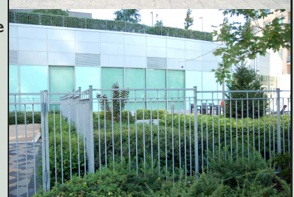
Bottom — Example of landscape planting surrounding parking ventilation
