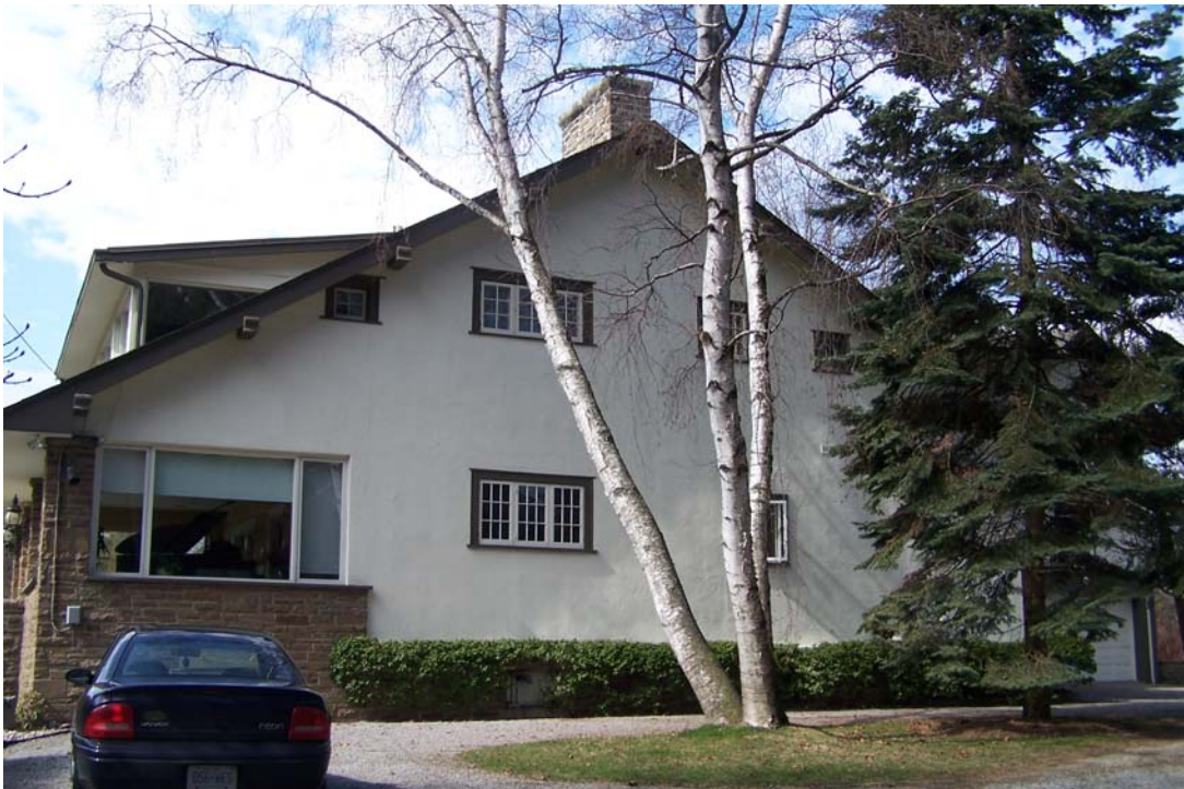
Figure 4: John A. Walker Cottage, east elevation
