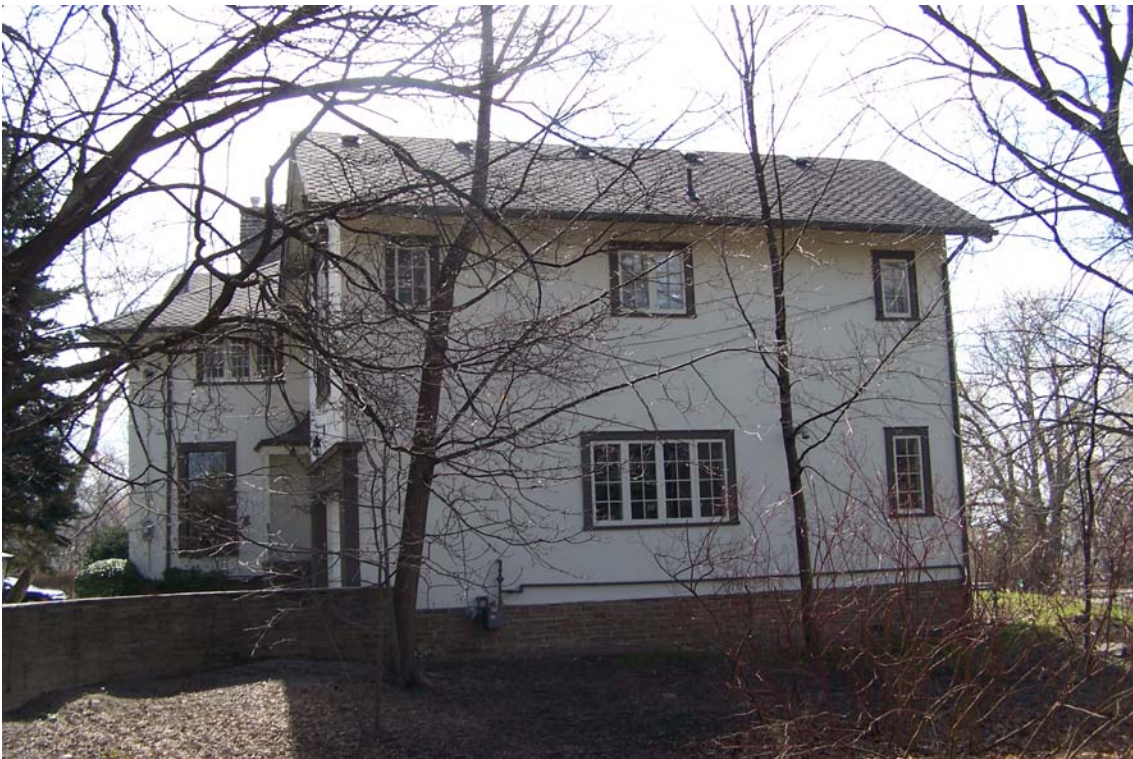
Figure 6: John A. Walker Cottage, north elevation
