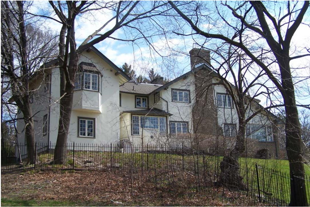
Figure 3: John A. Walker Cottage, view facing southwest
