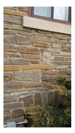
STONE DETAIL (NOTE CRACKING)
