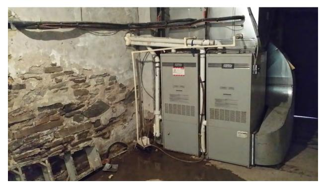
FURNACE ROOM (NOTE WALL DETERIORATION, STANDING WATER)
