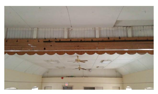
CEILING AT STAGE AREA (NOTE INADEQUATE FIRE PROTECTION)
