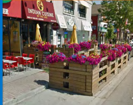
Parking Lay-by: Wooden Construction
