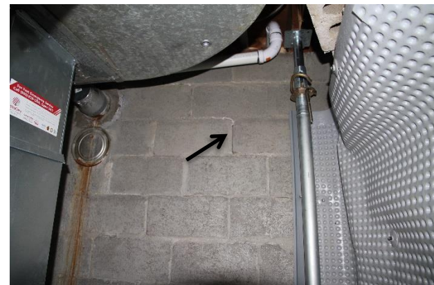
Figure 1 – Exterior view of the affected area, debris in the basement, and mortar cracks at the south wall.
