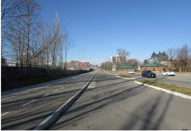
1. View looking northwest on Mississauga Road from parking lot of JC Saddington Park.
