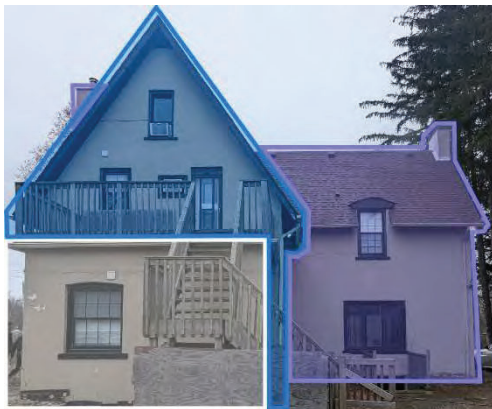
Photo #3: East Elevation, facing the backyard [JCAL 2024]
