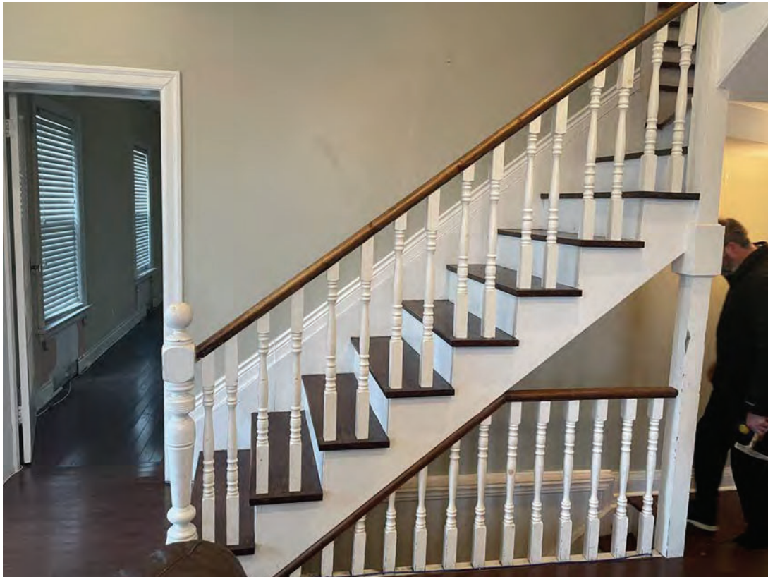
1 ST FLOOR STAIRCASE
