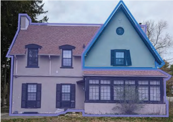
Photo #1: West Elevation, facing Clarkson Rd N [JCAL 2024]
