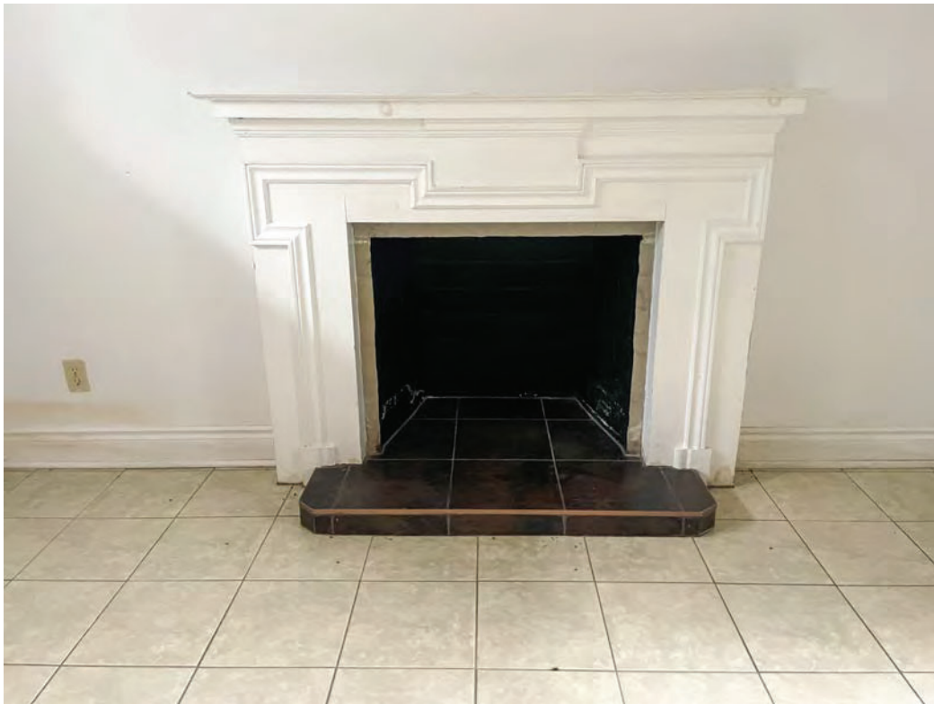
BASEMENT FIREPLACE WITH STONE OR CONCRETE SURROUND
