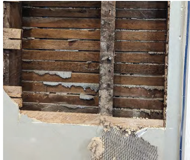
Photo #12: Interior partition wall construction between kitchen and living room [JCAL 2024]
