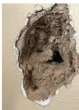
10" thick rammed earth walls
