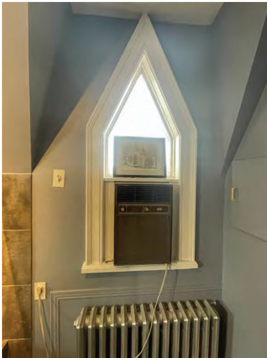
ORIGINAL POINTED WINDOW IN THE SIDE GABLE
