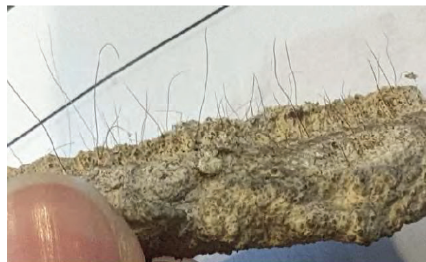
Photo #8: Animal hair observed in interior wall plaster, typical [JCAL 2024]
