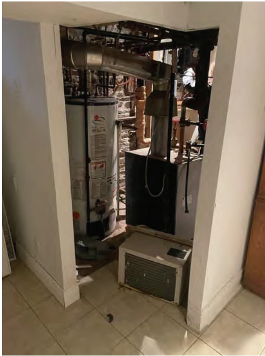
BASEMENT – FURNACE – IRREGULARLY COURSED STONE FOUNDATION WALL VISIBLE IN THIS AREA
