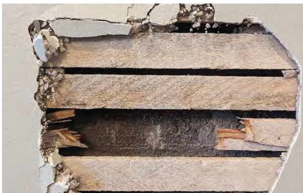
Photo #7: Horizontal wood lath, typical at interior face of walls [JCAL 2024]
