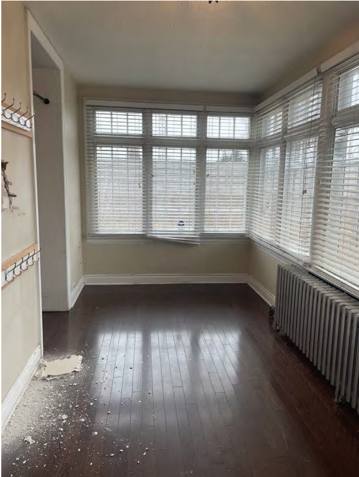
INTERIOR – FRONT SUNROOM TO BE REMOVED
