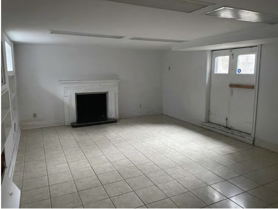
BASEMENT BELOW THE 2-STOREY ADDITION – TO BE DEMOLISHED
