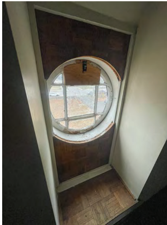
MODIFIED ROUND WINDOW IN THE FRONT GABLE
