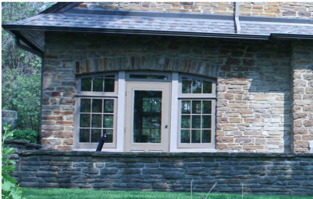
Figure 58 Detail of the stonework on the front façade. (Photo by author.)
