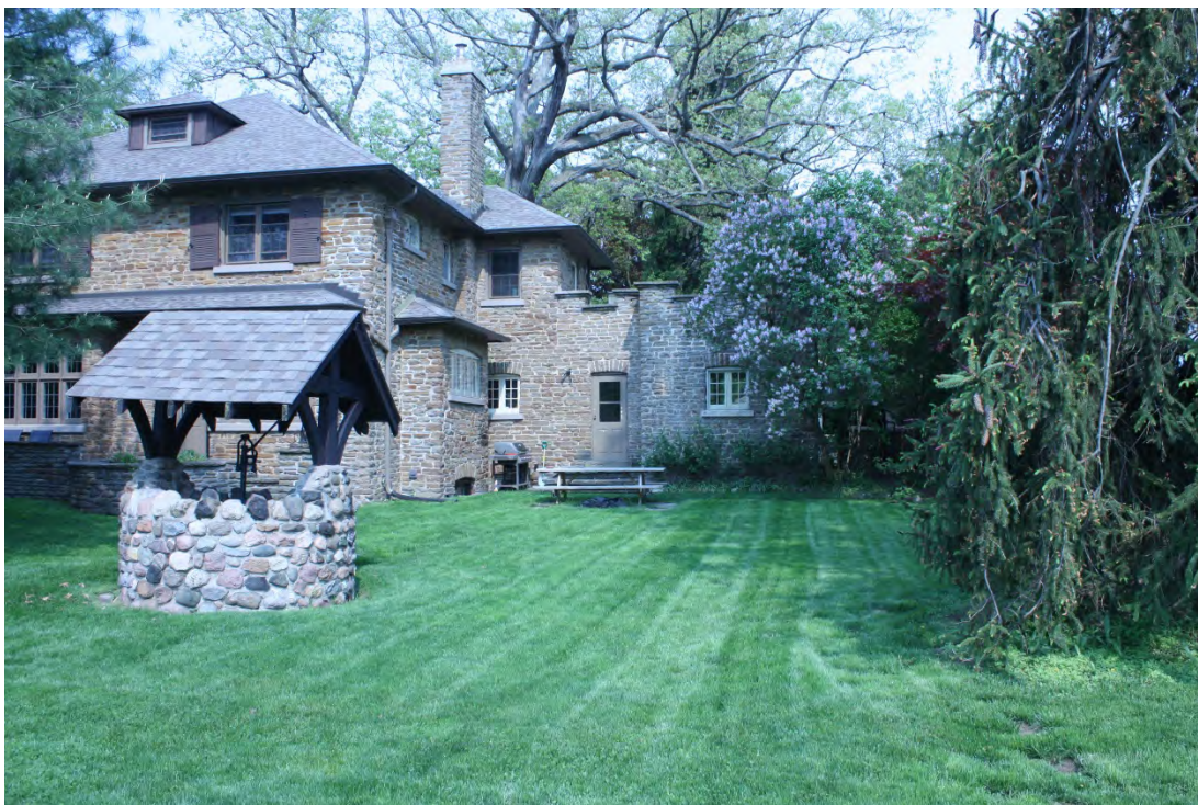
Figure 50 A wider view of the one storey portion of the structure proposed to be removed. (Photo by author.)
