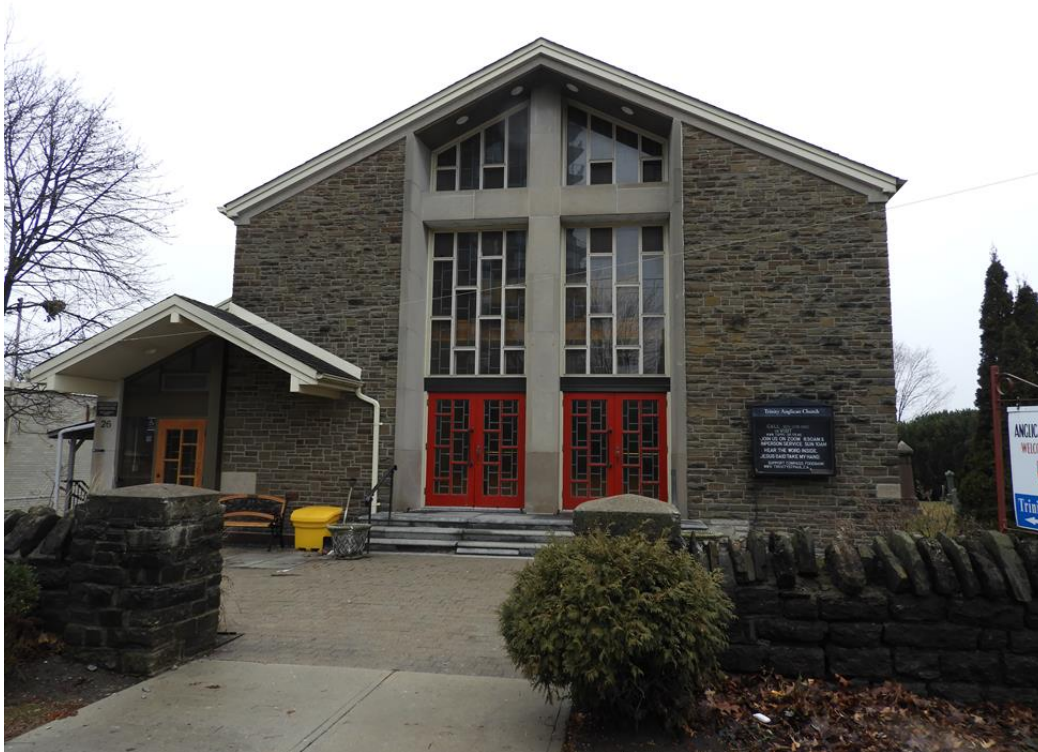
Front entrance view facing east
