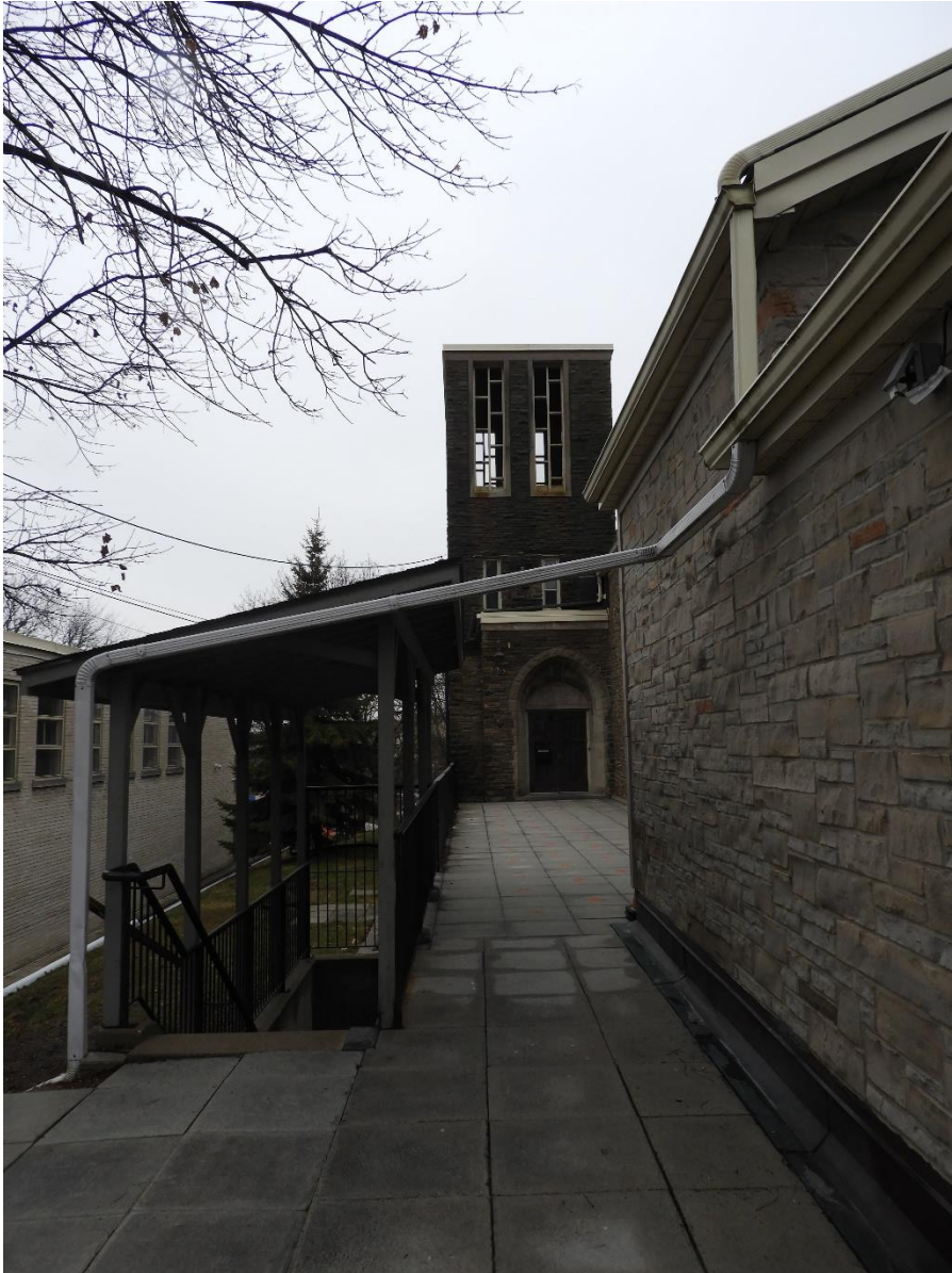
Tower from front
