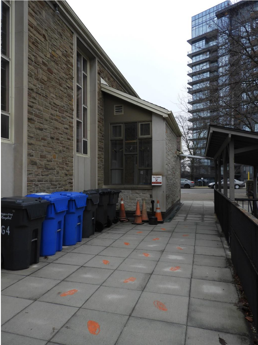
2001 addition facing east (standing in front of the tower)
