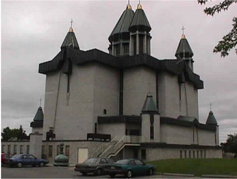
Photographs from Heritage Designation Statement ca. 1980
