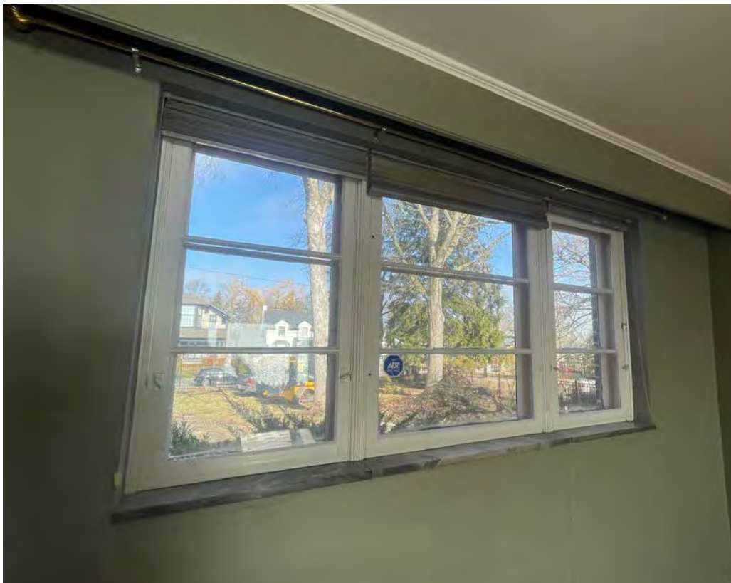
FRONT ELEVATION – WOOD CASEMENT WINDOWS
