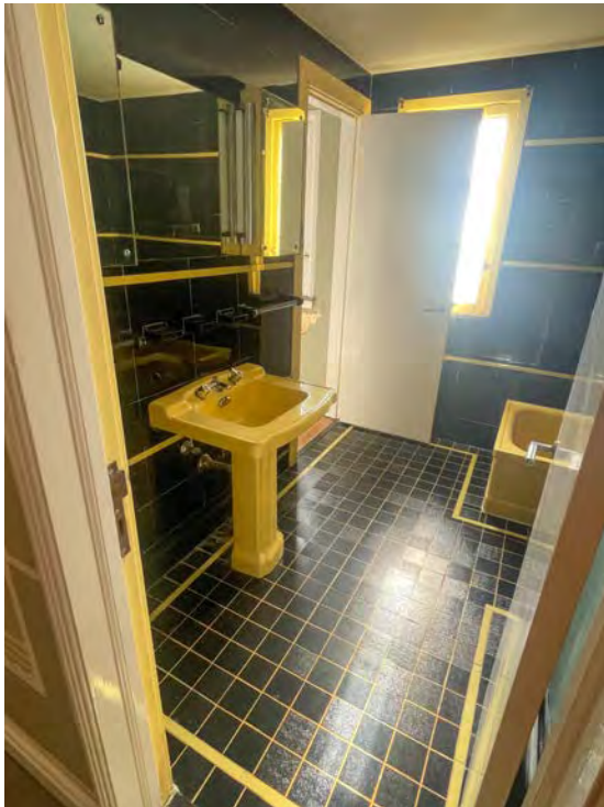
INTERIOR – 2 ND FLOOR - BATHROOM
