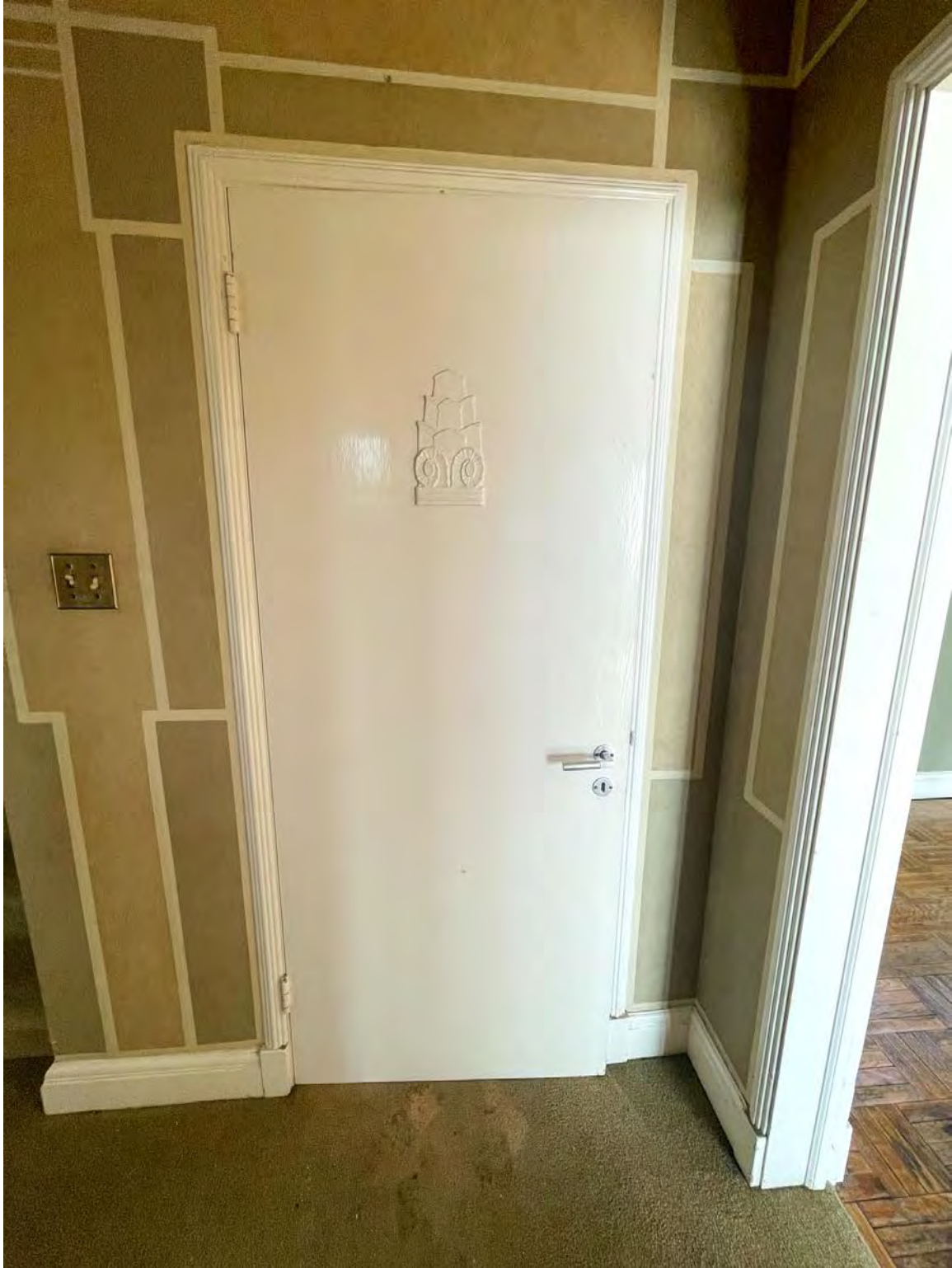
INTERIOR DOORS & ORIGINAL HARDWARE
