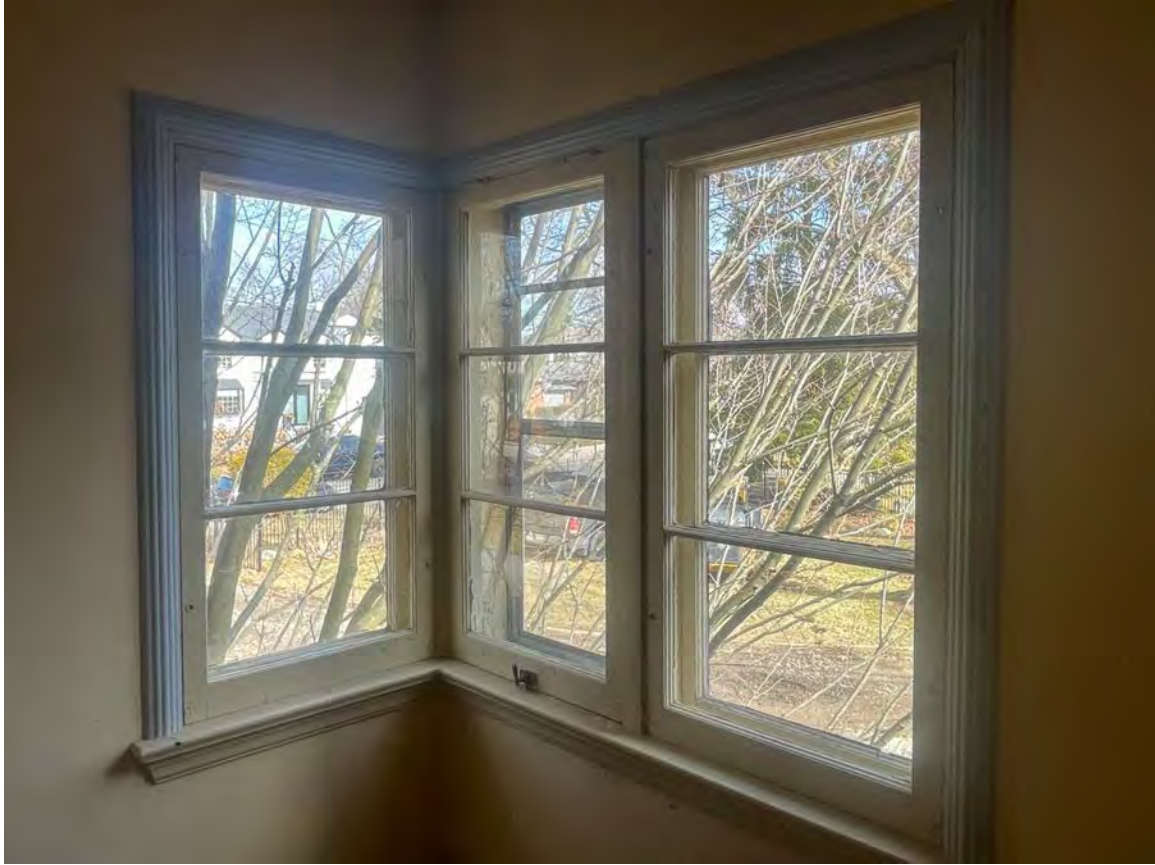
INTERIOR - GARAGE – 2 ND FLOOR - BEDROOM – corner window
