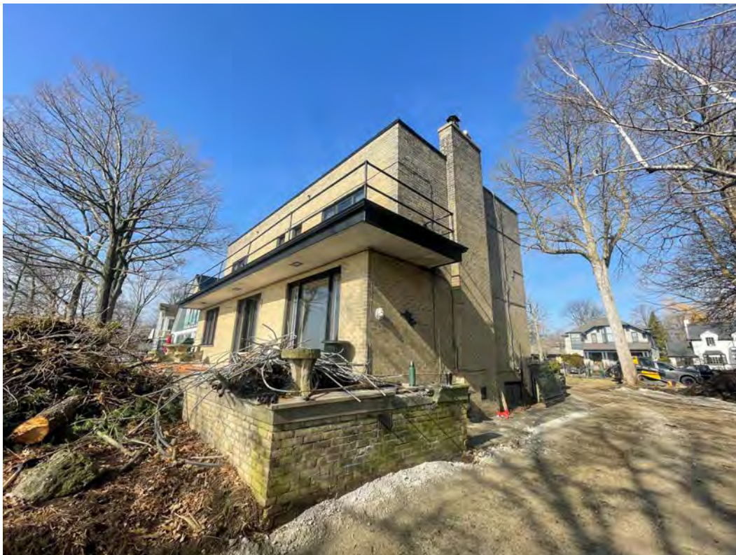
SIDE & REAR ELEVATION – cantilevered balcony with metal railings on the rear elevation
