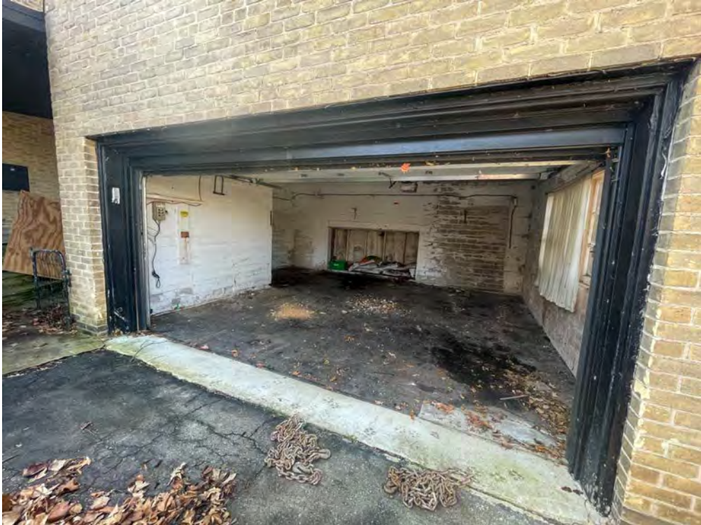
GARAGE INTERIOR – 1 ST FLOOR
