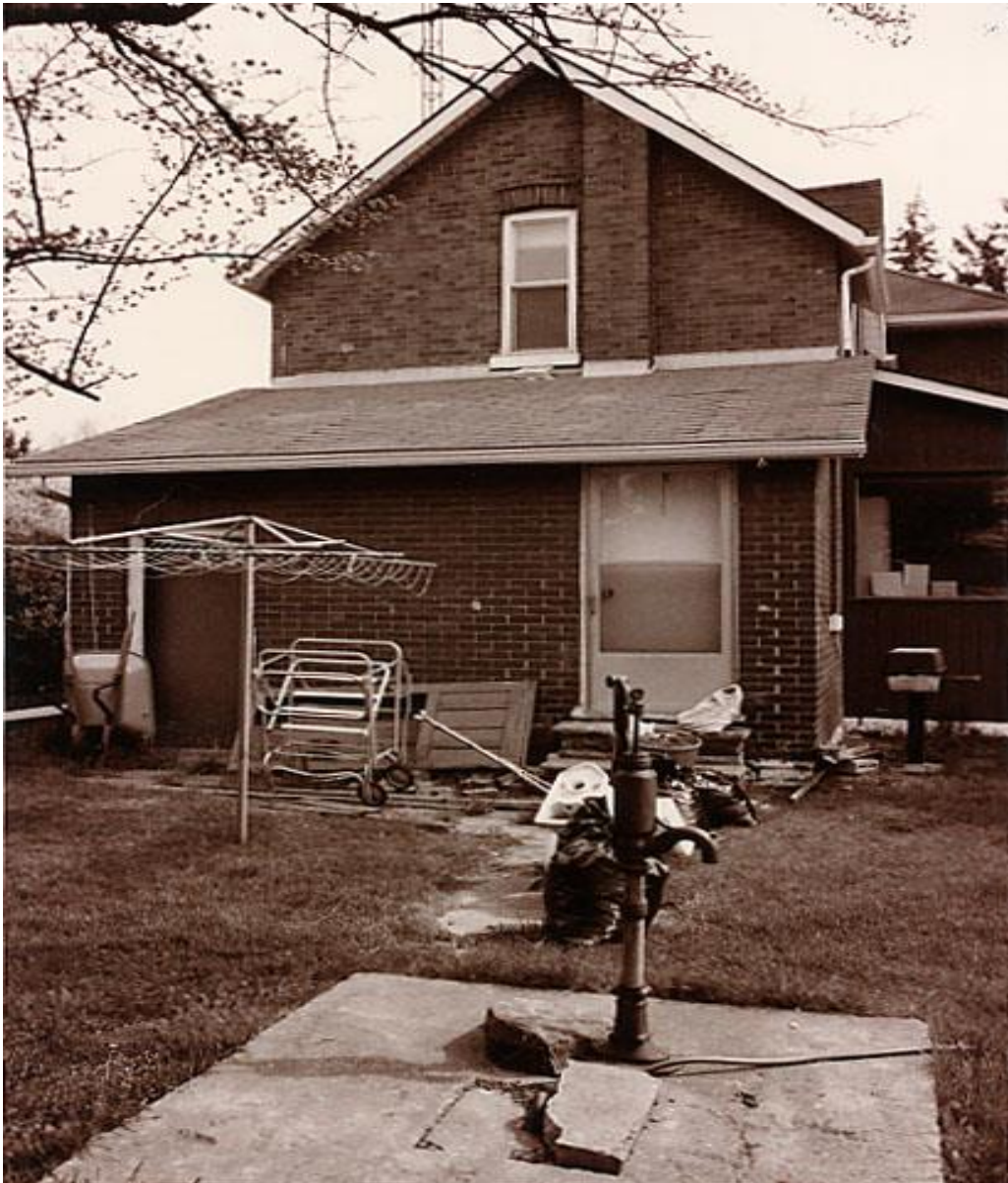
Image dated 1989; west façade of house with pump in foreground
