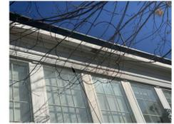
NOTE DETERIORATED AND LEAKING SOFFIT. THIS IS EXPECTED TO BE CAUSED BY LEAKAGE IN THE CONCEALED GUTTER ABOVE
