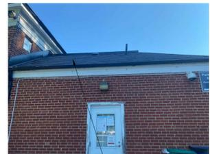
NOTE DETERIORATED SHINGLES AT LOWER ROOF
