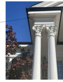
NOTE DETERIORATED SOFFIT AT ENTRY PORTICO. THIS IS LIKELY CAUSED BY LEAKING OF CONCEALED GUTTER ABOVE
