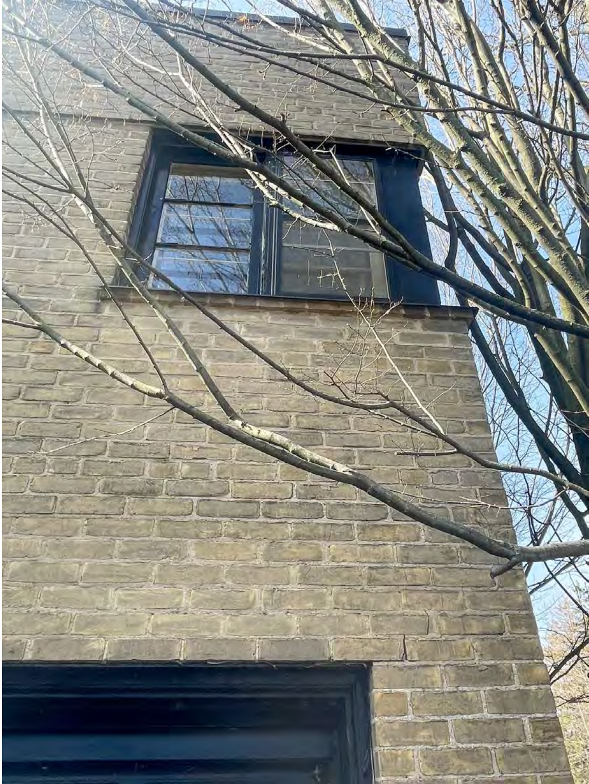
GARAGE – corner window
