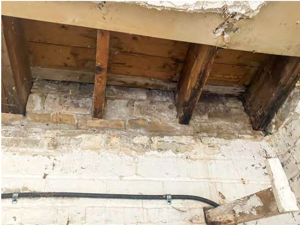
GARAGE INTERIOR – 1 ST FLOOR – concrete block walls with wood framing above
