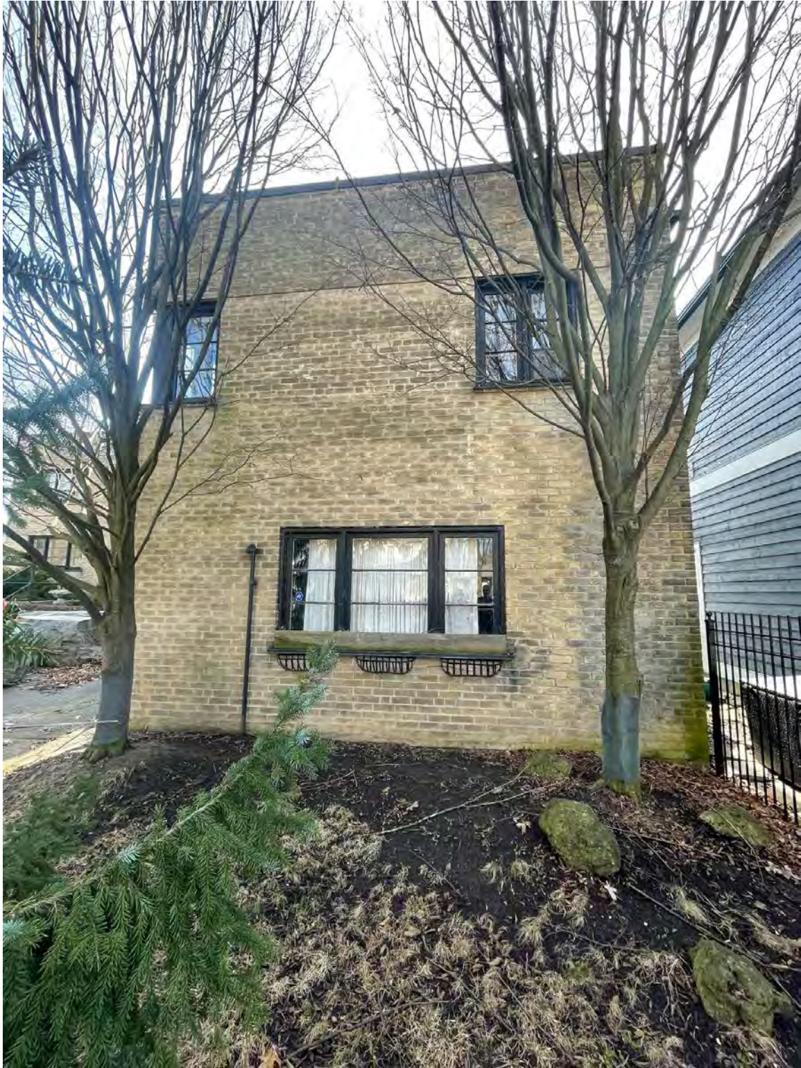
GARAGE – wood casement windows
