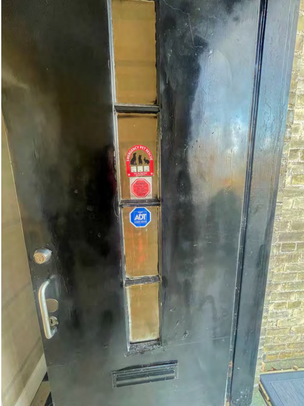
FRONT ENTRANCE DOOR – WOOD WITH GLAZING
