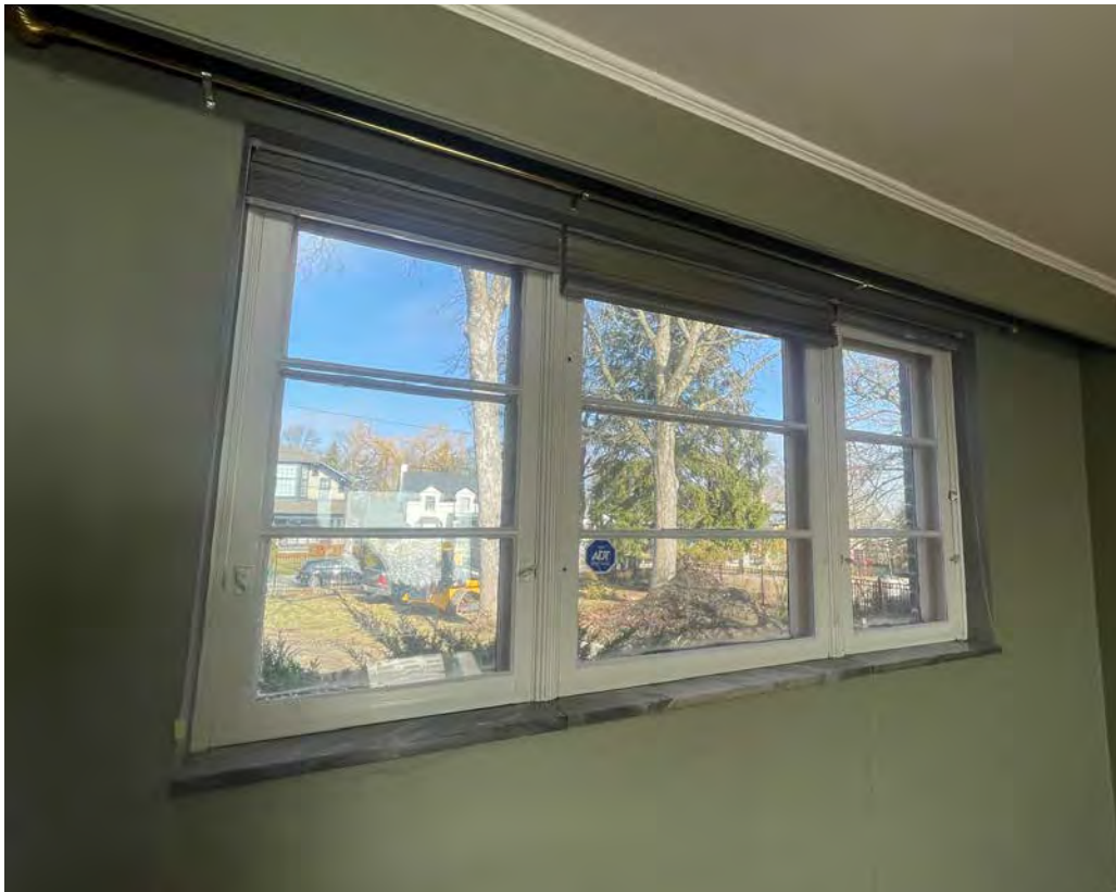
FRONT ELEVATION – WOOD CASEMENT WINDOWS
