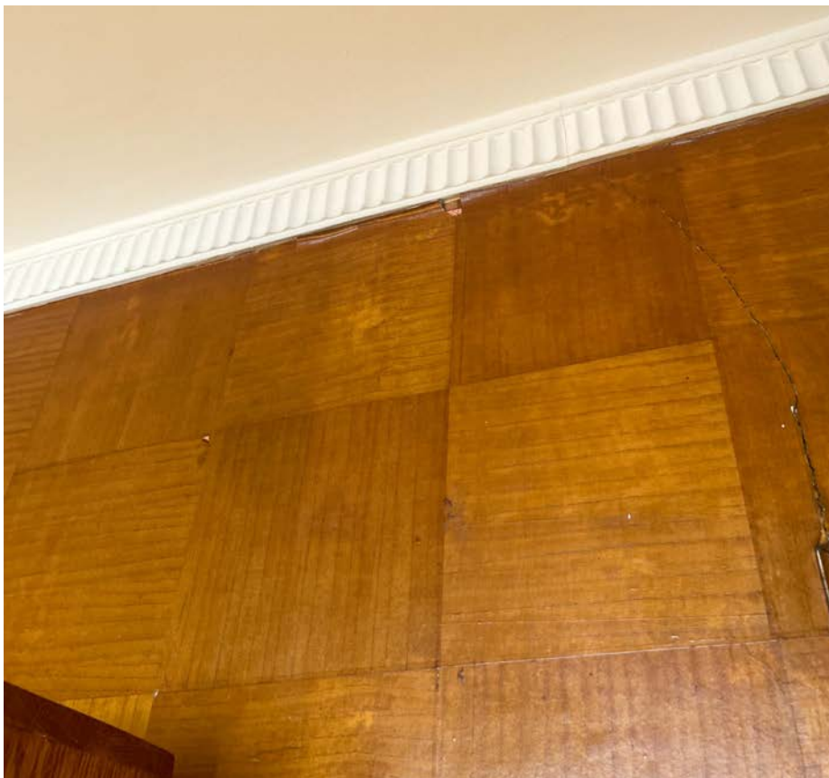
WOOD WALL PANELING
