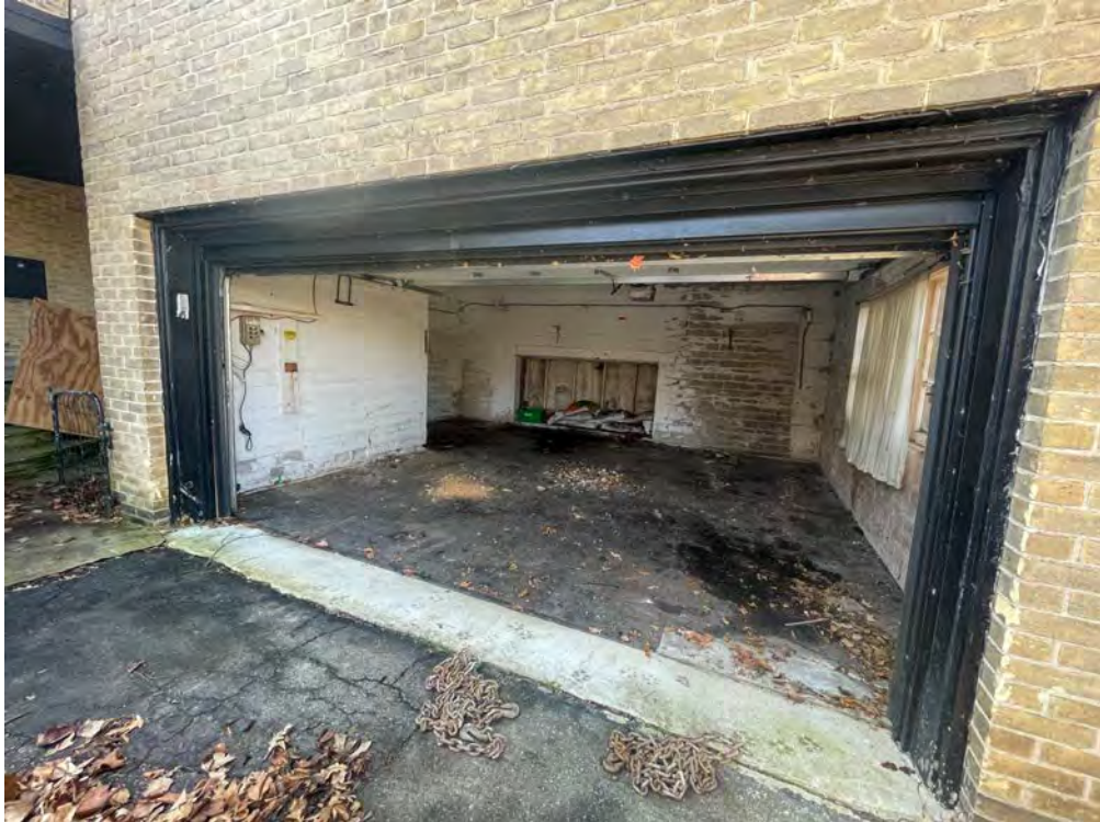
GARAGE INTERIOR – 1 ST FLOOR
