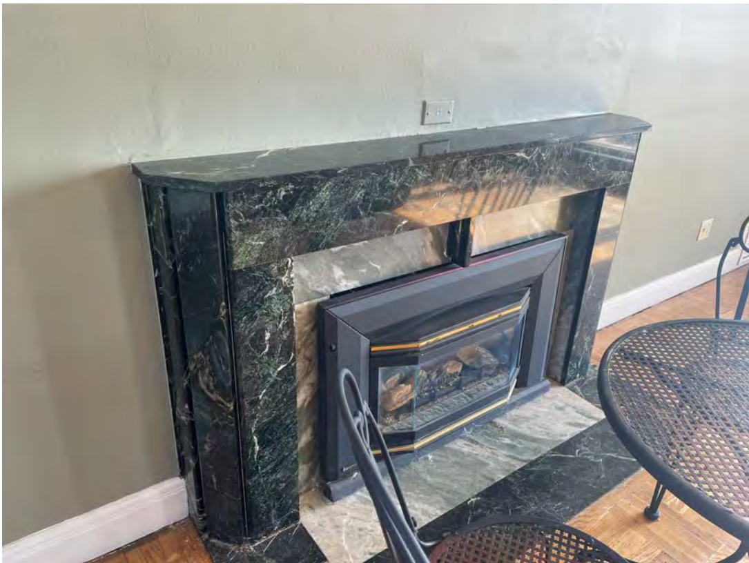
INTERIOR – 1 ST FLOOR - FIREPLACE
