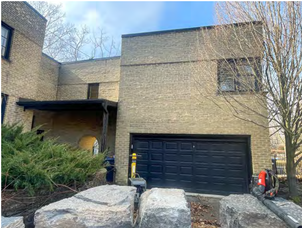
GARAGE & LINK STRUCTURE – note the 2 nd floor corridor linking the house and garage and the brick arch below with an iron gate to the side yard
