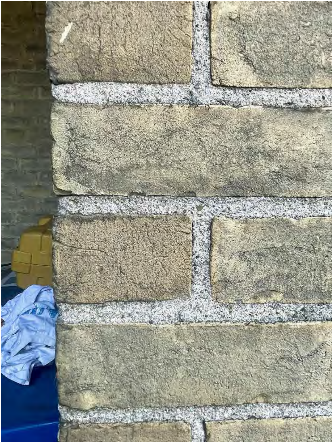
BUFF BRICK – salvaged brick can be used as a repair material
