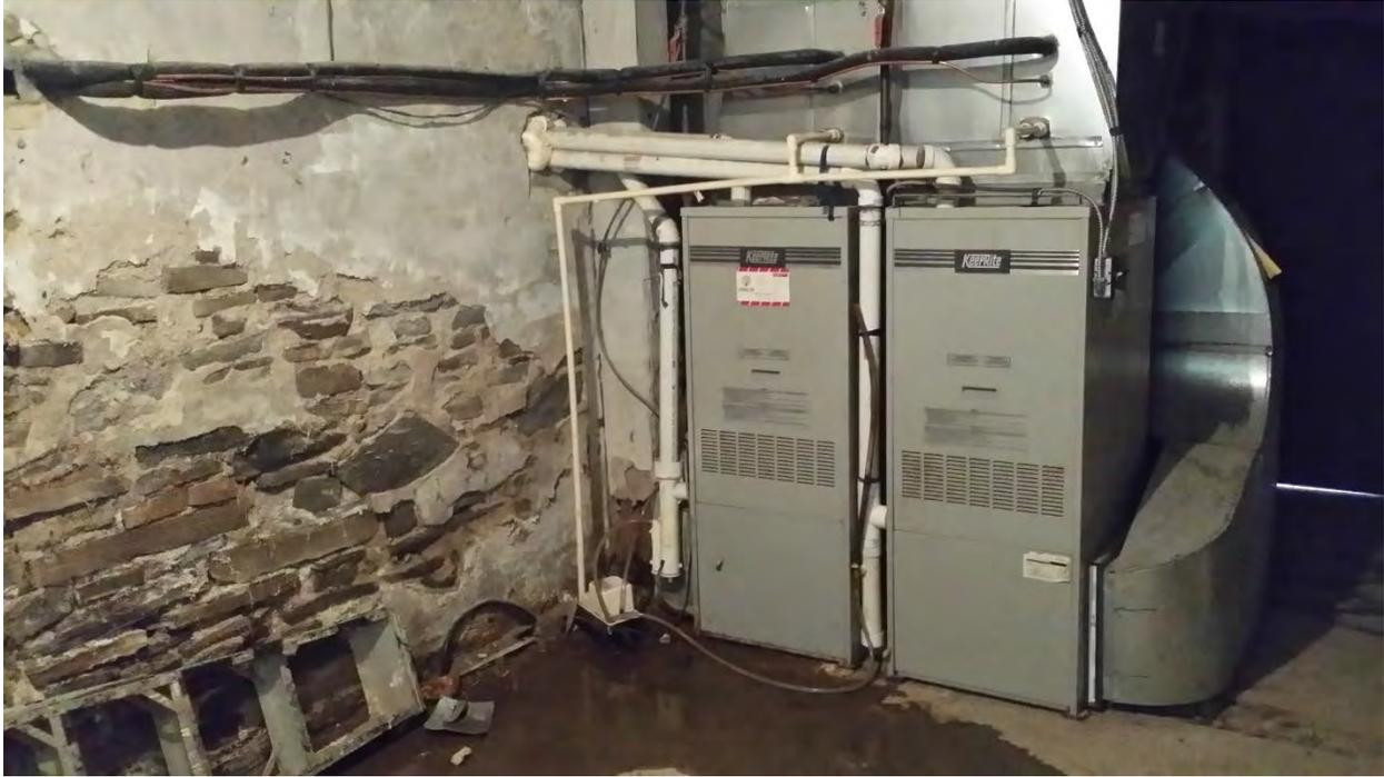
FURNACE ROOM (NOTE WALL DETERIORATION, STANDING WATER)
