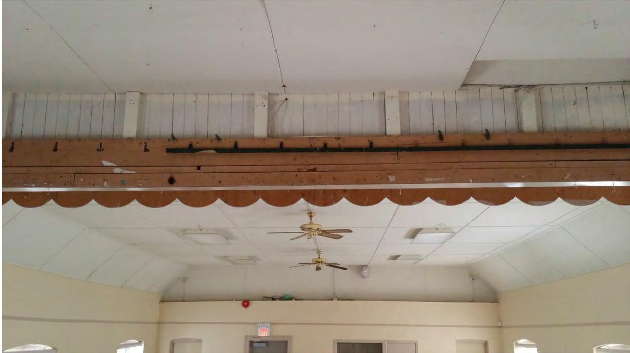
CEILING AT STAGE AREA (NOTE INADEQUATE FIRE PROTECTION)
