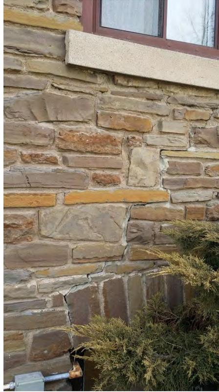
STONE DETAIL (NOTE CRACKING)
