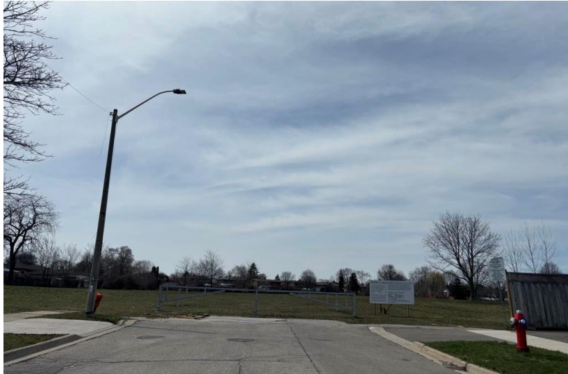
Figure 2: Property Condition, Photographed April 11, 2024
