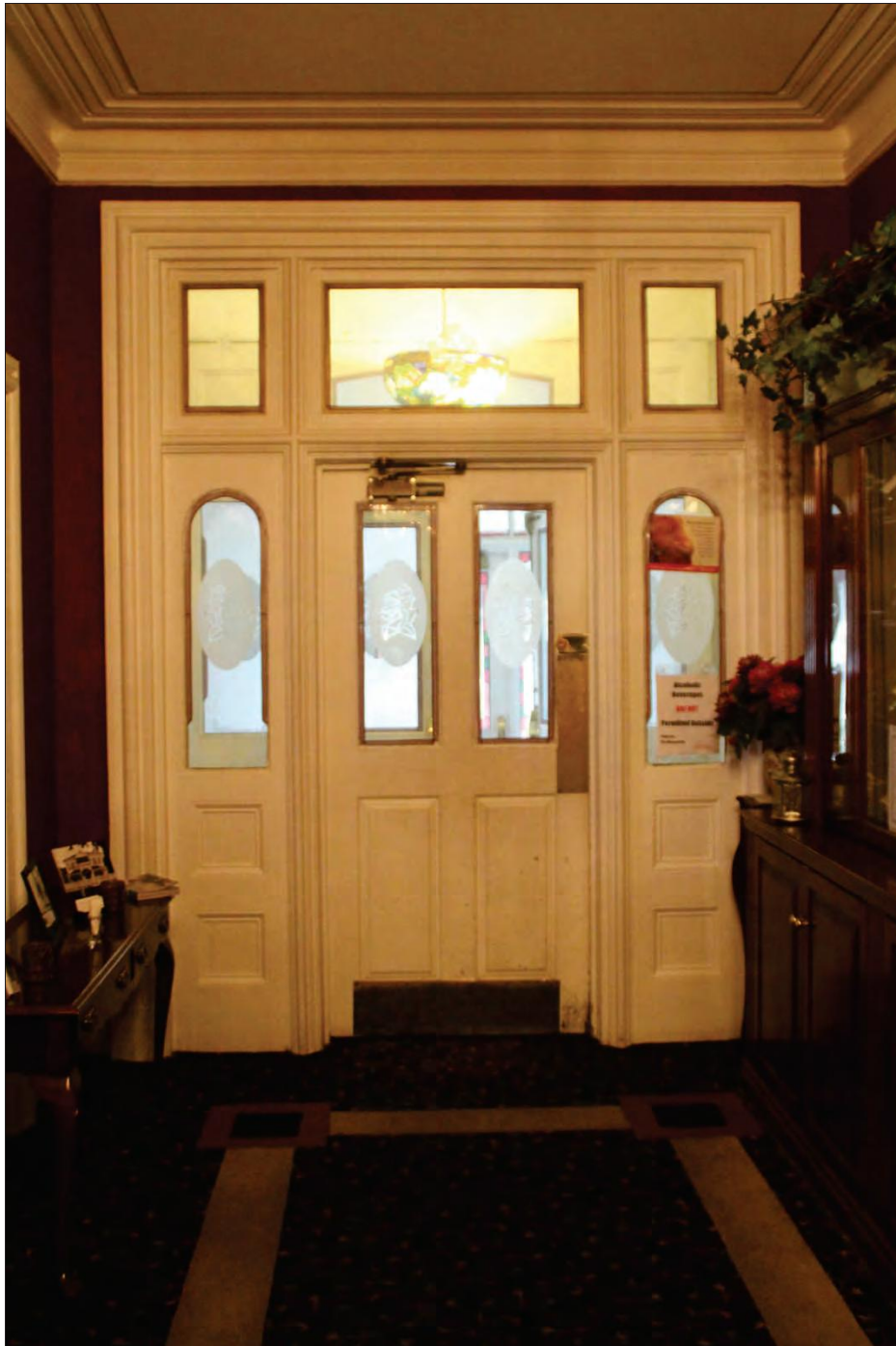
Figure 41 inside front door, transom & sidelights (replacement glass), ceiling moulding
