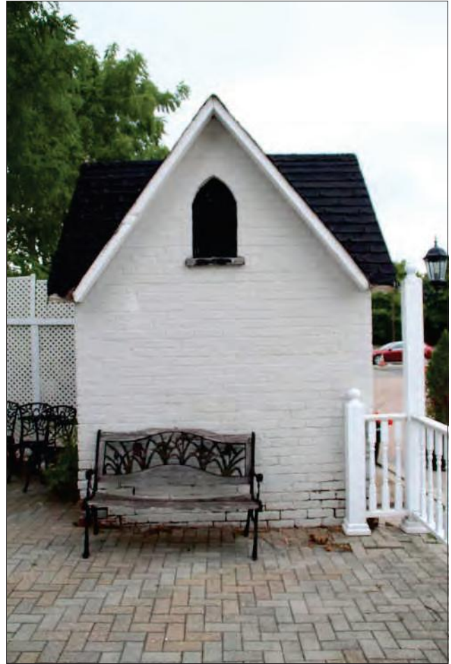
Figure 60 outbuilding - west facade
