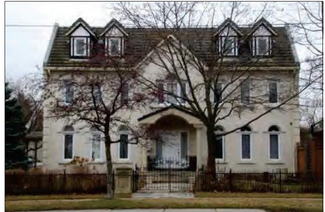
Fig 64 west side Mississauga Rd-opposite subject property
