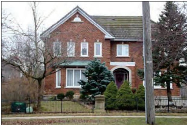
Fig 65 west side Mississauga Rd-opposite subject property
