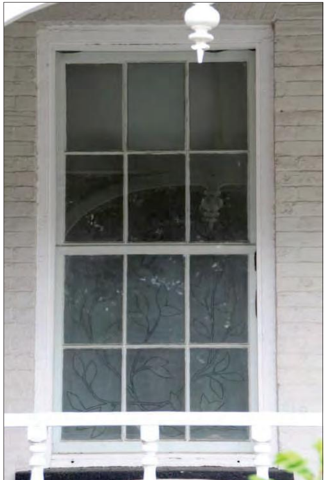
Figure 376 typical 6/6 sash window
