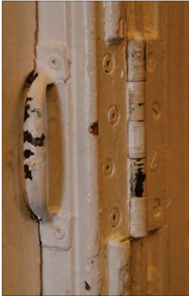
Figure 48 pocket door hinge & handle
