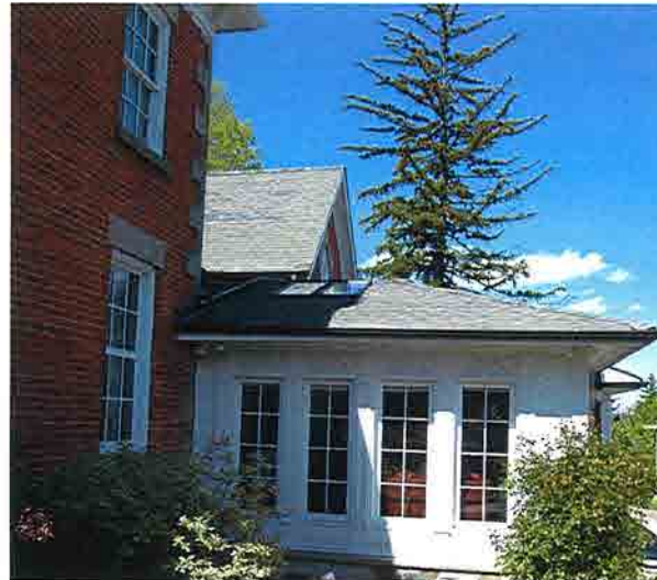
5. The addition on the south side of the building.
