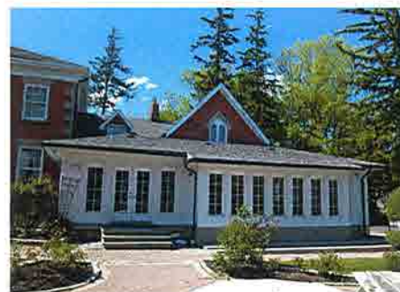
The photo above shows the finished addition. The materials used complement the existing building rather than clashing with it. Steps were taken so architectural elements of importance in the original house wouldn't be destroyed or obscured by the addition; such as the round headed window seen in this photo above the addition.
