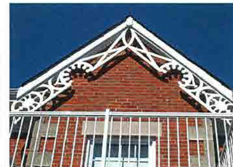
Vergeboarding on gable end at the front of the house.
