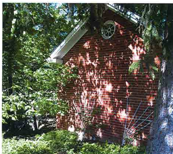
12. Round window on the west elevation of the outbuilding
