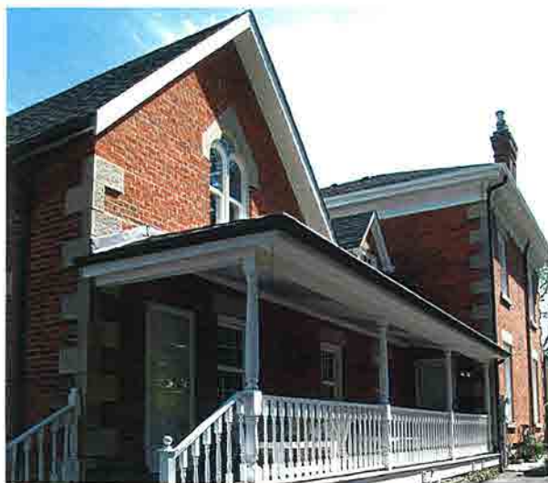
14. Rounded windows with triangular carved stone lintel on the house
