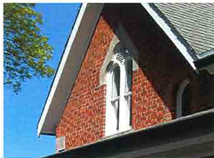
Round headed window and rounded louver with triangular carved stone lintel.
