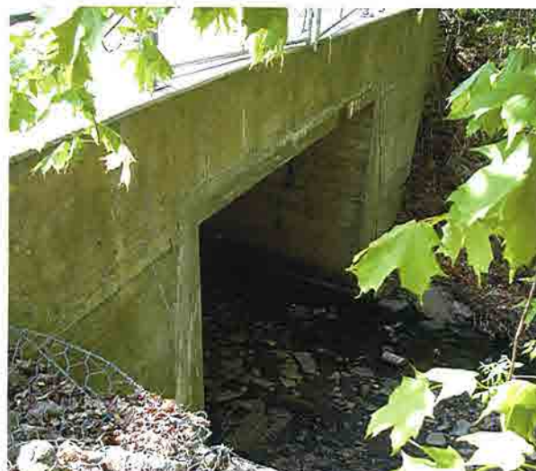
27. Storm drain as it passes under Hammond Road, unlike the one at the east end it has no cage.
