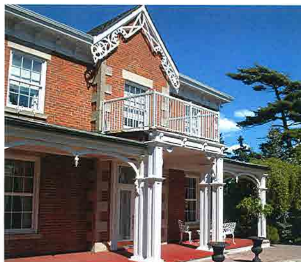
2. Recessed front door from the 50's was replaced by flush, glazed double doors.
