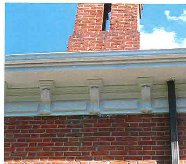
25. Brackets below the roof.
