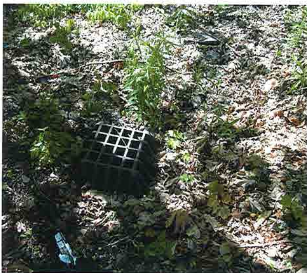
20. Catch basin located near where the creek meets King Forest Drive.
