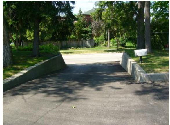
Looking west to Hammond Road: concrete embankment wall and asphalt driveway.
