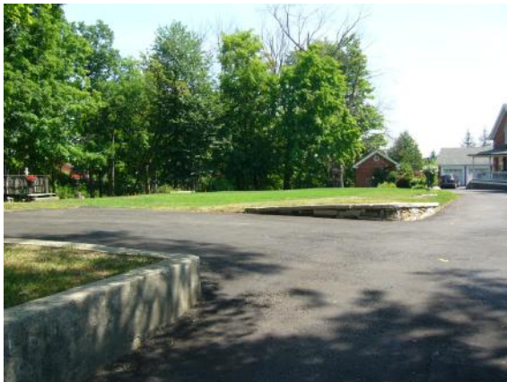
Looking east: concrete embankment, asphalt parking pad, asphalt driveway and low stone wall.
