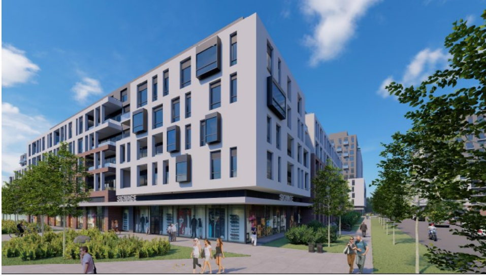
BUILDING E (view looking southwest from Ninth Line & Street B)
