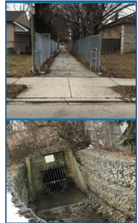
Malton Drainage Improvements
