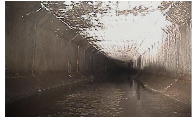
Storm sewer Improvements
