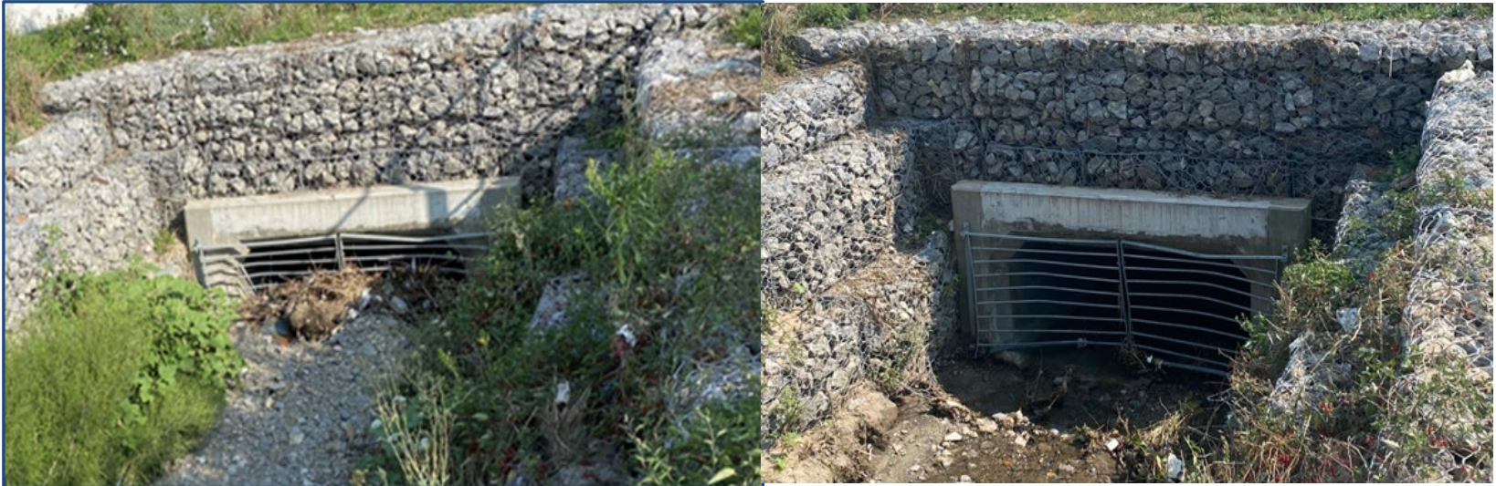
Inlet North of The Queensway
