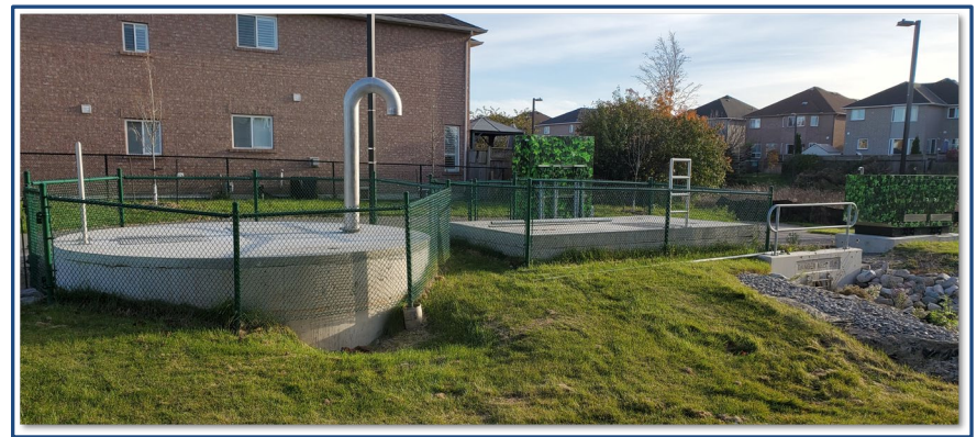
Cactus Gate Pumping Station
