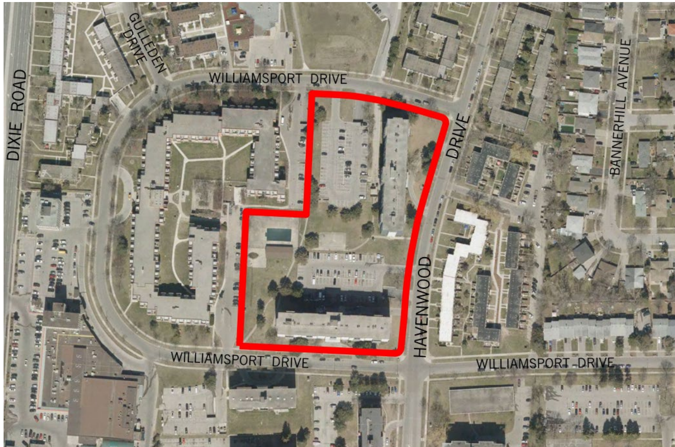
Aerial Photo of 1485 Williamsport Drive and 3480 Havenwood Drive
