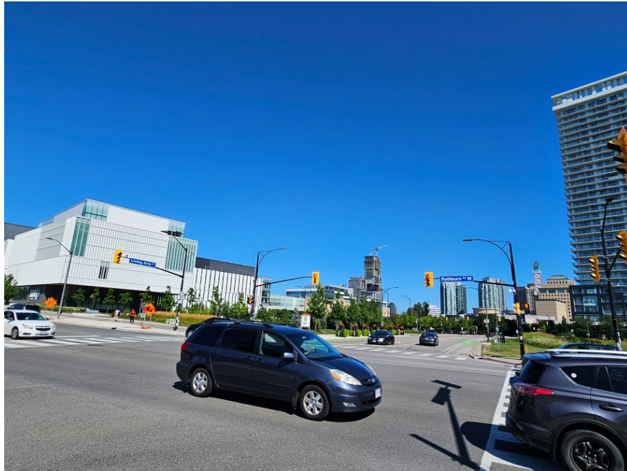
Lands to South at Rathburn Road West and Living Arts Drive (facing south)
