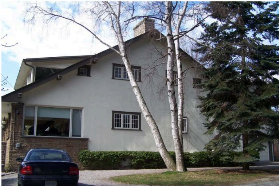
Figure 4: John A. Walker Cottage, east elevation
