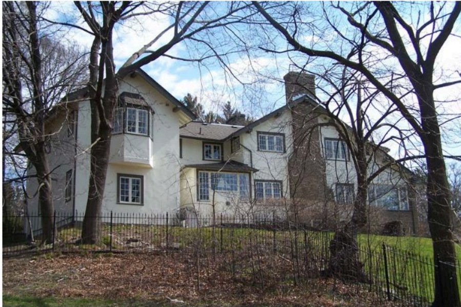
Figure 3: John A. Walker Cottage, view facing southwest
