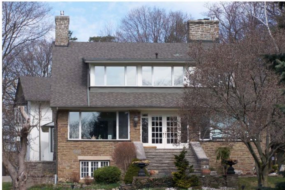
Figure 2: John A. Walker Cottage, south façade
