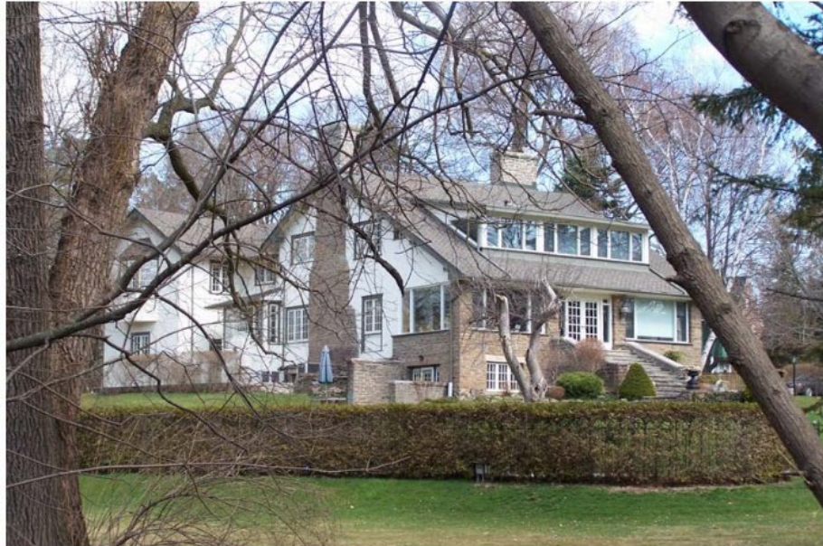
Figure 1: John A. Walker Cottage, view facing northeast
