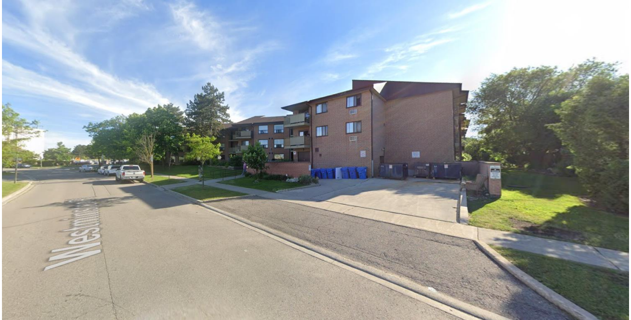
Photo of Existing Site Condition (view looking west from Westminster Place)
