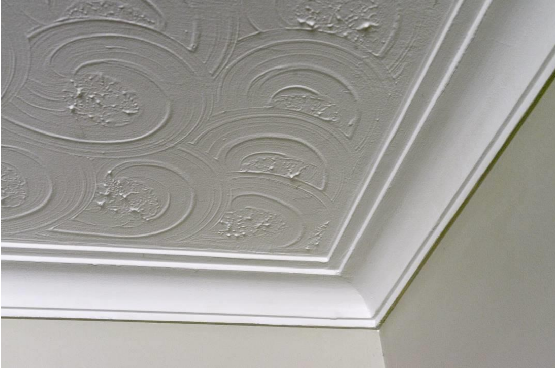
Fig. 31 Plaster ceiling and cornice (crown moulding) in combination living and dining room
