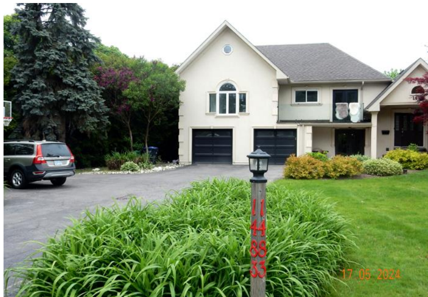
Figure 21: 1483 Mississauga Road, LDW
