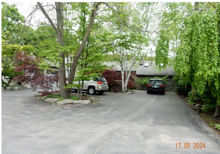
Figure 5: 1495 Mississauga Road Looking North from Sidewalk, LDW
