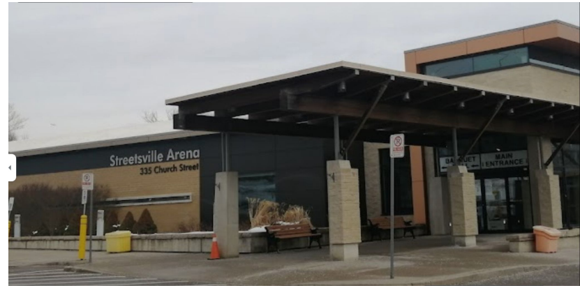
Vic Johnston Community Centre
