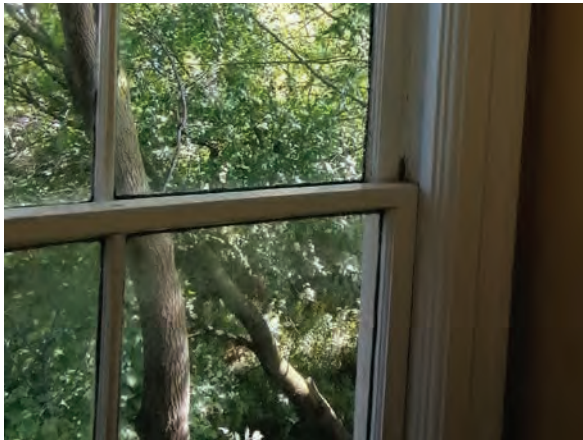
Detail of east elevation second storey window and trim showing cut sash cord (ERA, 2021).
