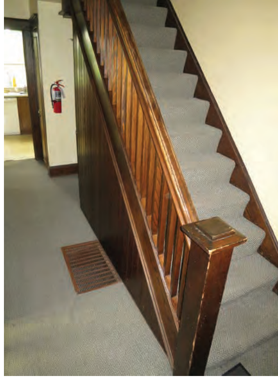
Staircase from first floor (ERA, 2022).
