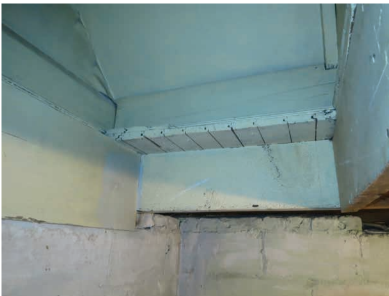
Underside of main staircase from basement stairs (ERA, 2022).
