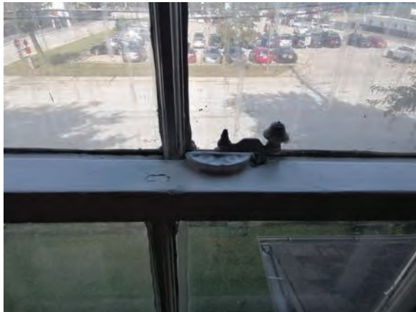
Detail of north elevation second storey window showing sash lock (ERA, 2021).
