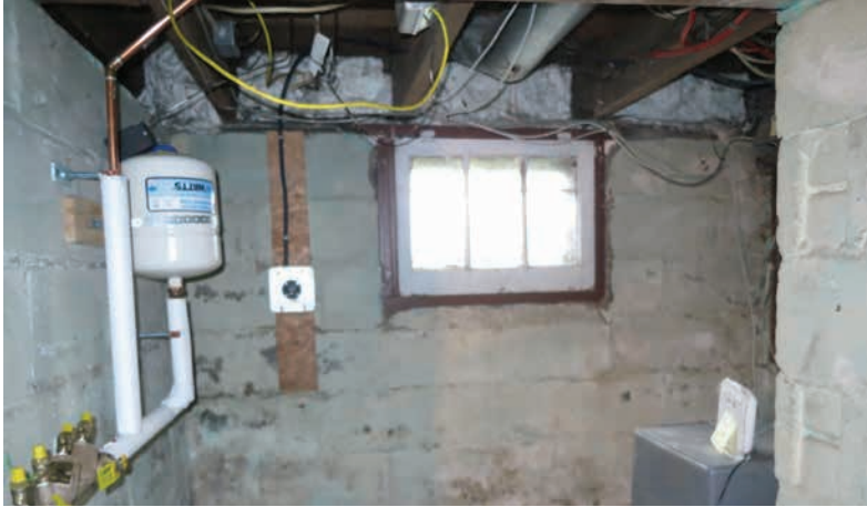
Foundation wall, not thinness compared to previous image (ERA, 2022).
