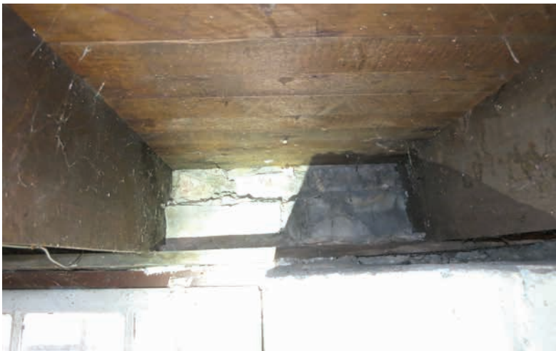
Top of foundation wall (ERA, 2022).
