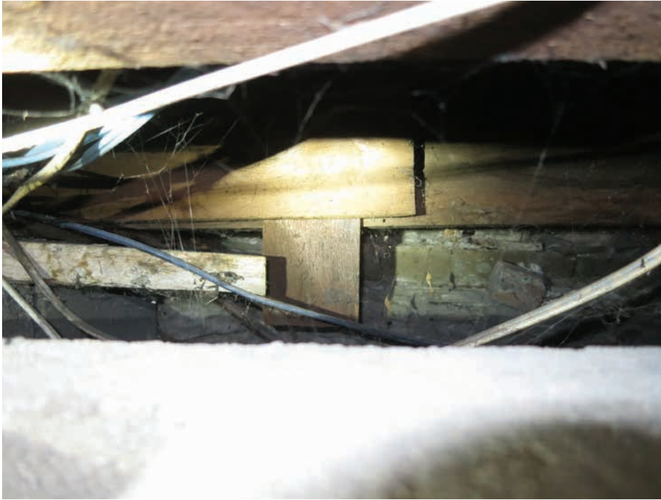
Exposed rubble foundation wall (ERA, 2022).
