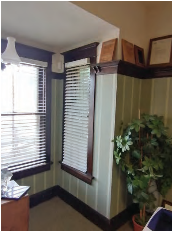
First floor bay-window, wood trim and plate rail (ERA, 2021).
