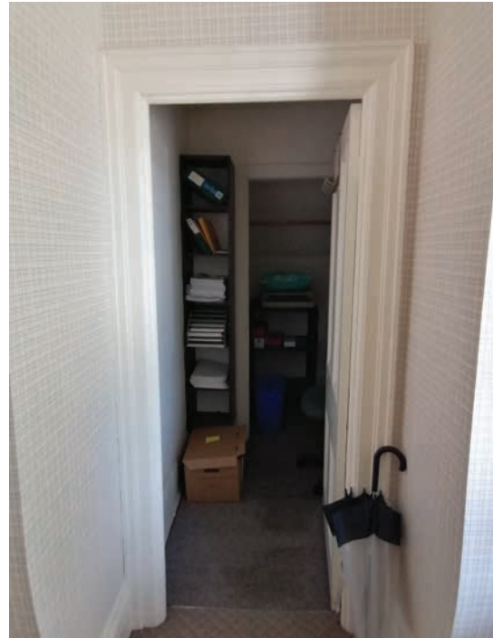
Second floor wood trim (ERA, 2021).
