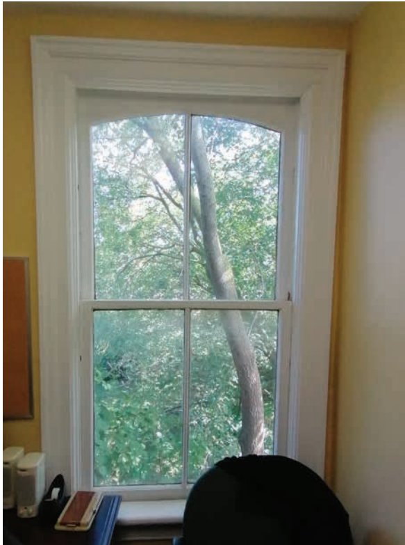
East elevation second storey window and trim (ERA, 2021).
