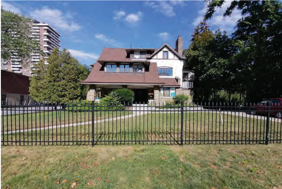
South elevation of 84 High Street East (ERA, 2021).
