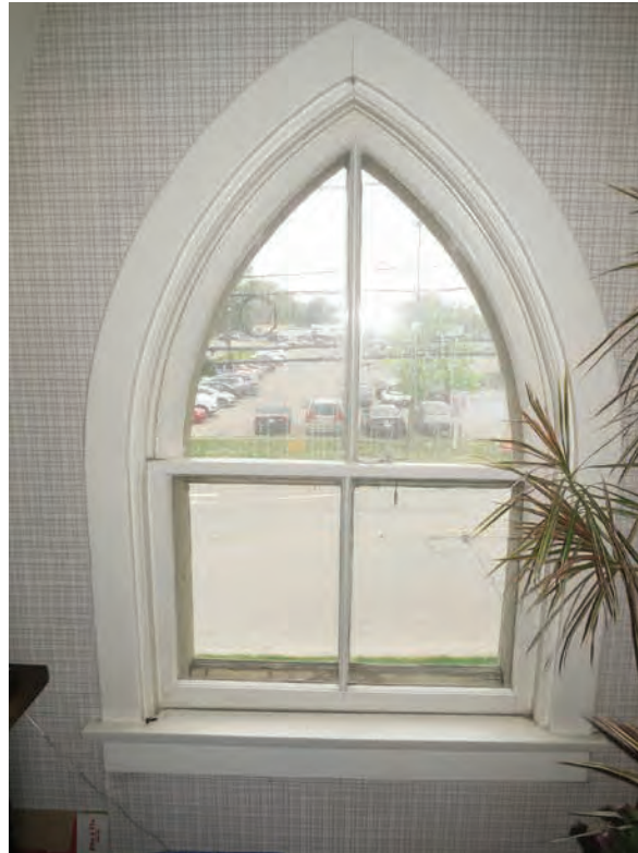
North elevation second-storey lancet window (ERA, 2022).
