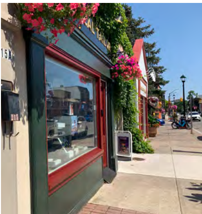
Commercial buildings along Queen Street South.
