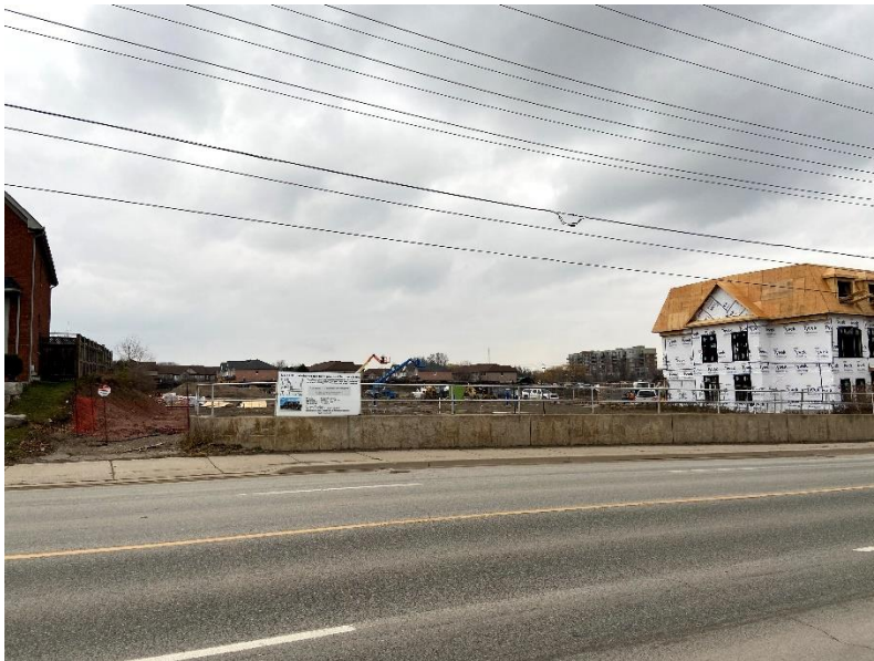
Image of existing condition facing north
