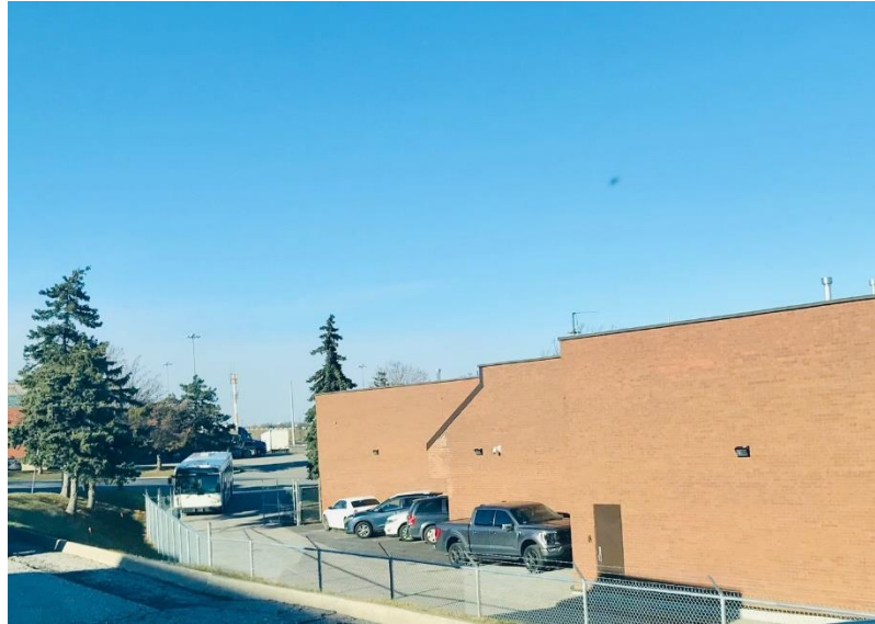
Photo 1: Vehicles parking at side of building. Accommodates 5 vehicles, not shown on Site Plan.
