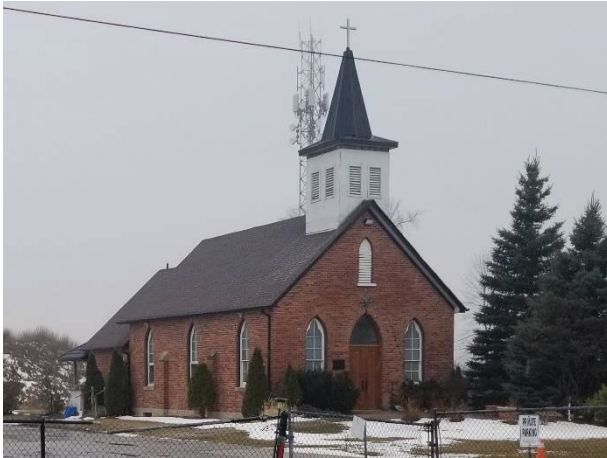
Plate 10: Oblique view of the east and south elevations.
