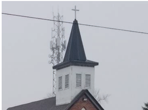
Plate 13: South and east elevations of the bell tower.
