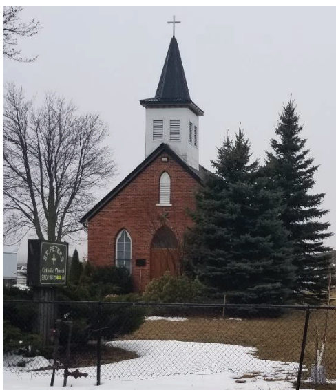
Plate 6: Front (east) elevation.
